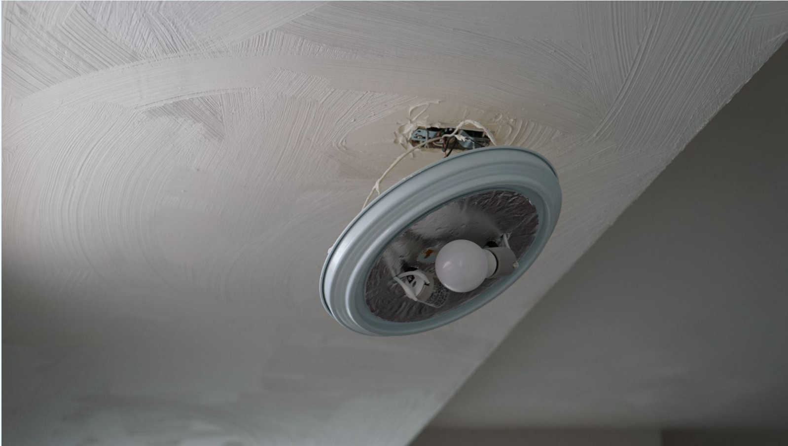
Above: Damaged light fixture pulled away from the ceiling
