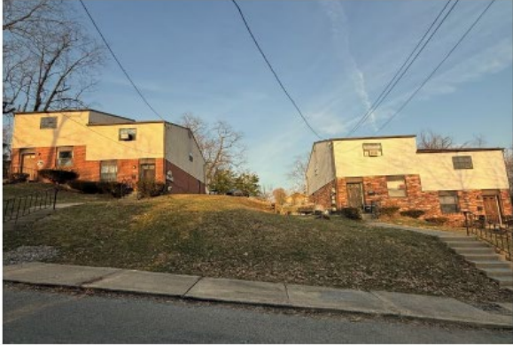
A: West Elevation Front Façade
