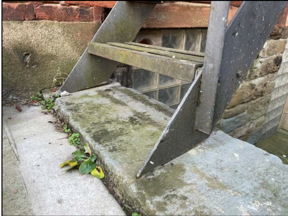
Photo 1. Missing Stair Base Attachment
