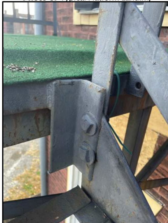
Photo 6. Typical Stair Stringer Attachment to Landing
