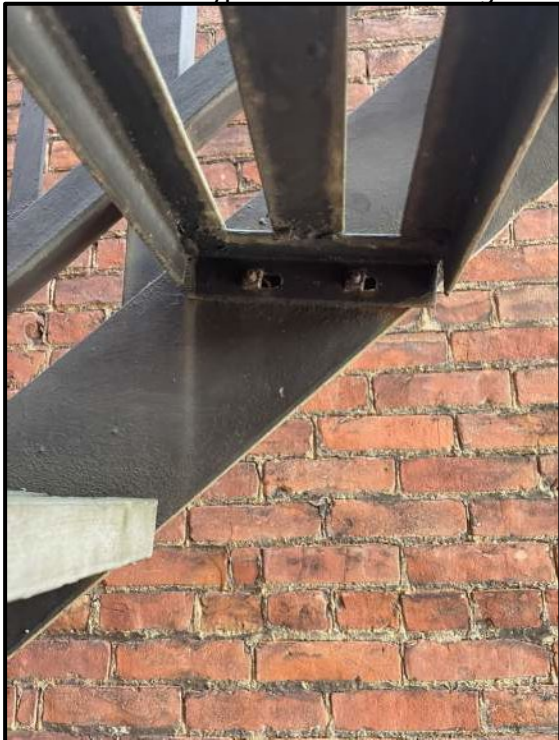
Photo 6. Typical Stair Tread Attachment to Stringer
