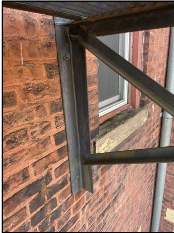
Photo 3. Typical Platform Brace Connection
