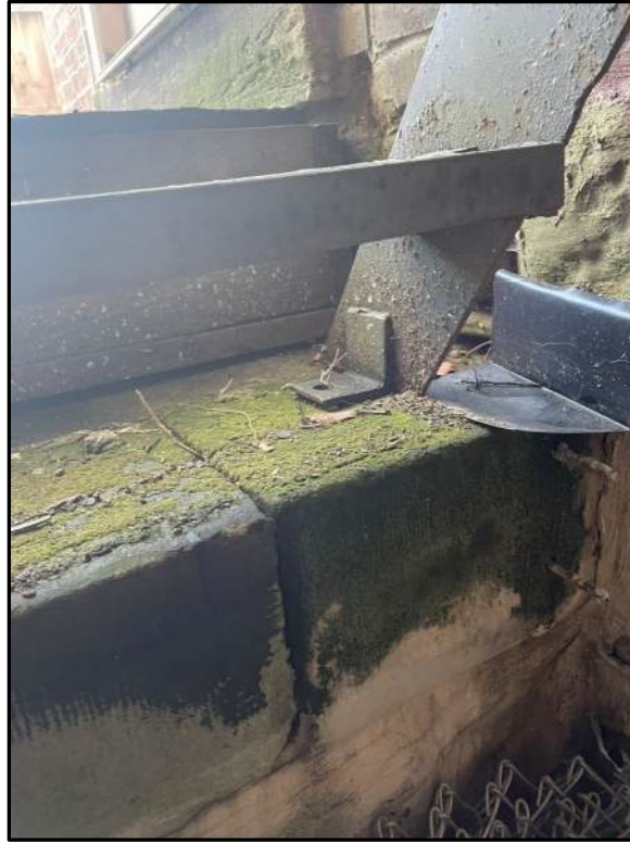
Photo 1. Missing Stair Base Attachment
