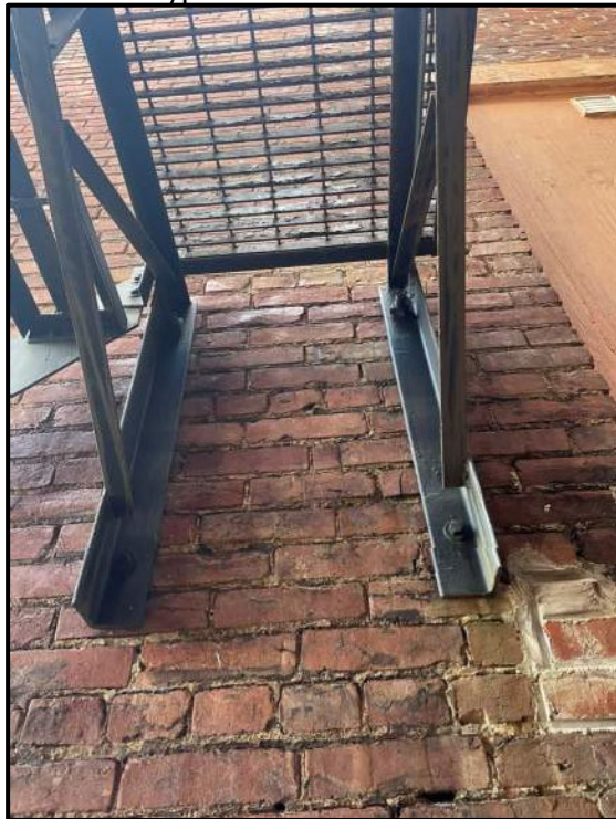
Photo 4. Typical Platform Brace Connection
