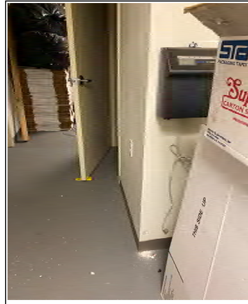
Photograph No. 10– Wall plaster in basement
