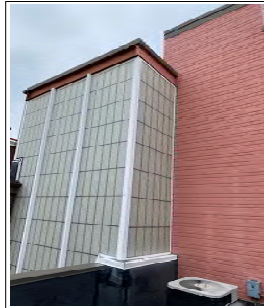
Photograph No. 38 – View of the building
