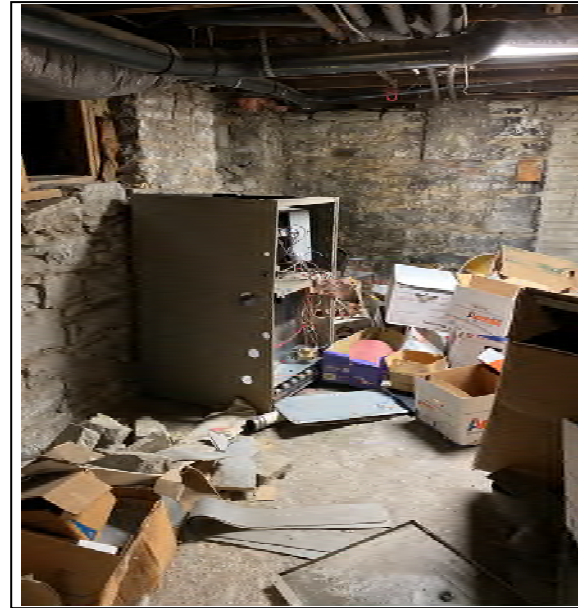
Photograph No. 8 – Basement
