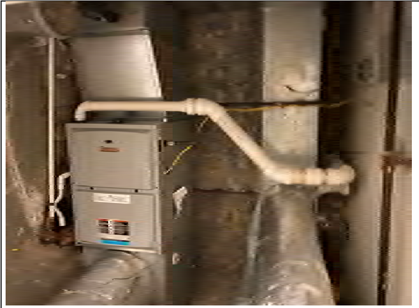
Photograph No. 9– Pipe insulations
