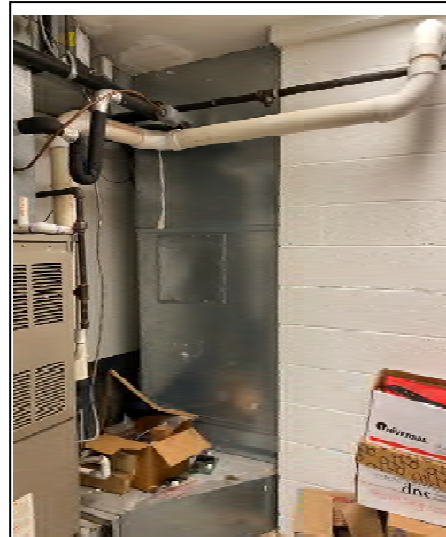
Photograph No. 16 – Wall paint and plaster
