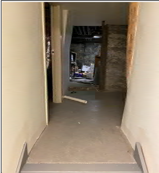
Photograph No. 7 – Basement
