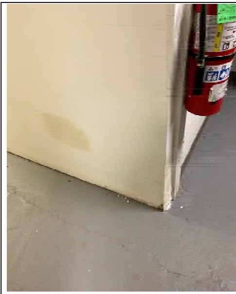
Photograph No. 11 – Wall plaster in basement
