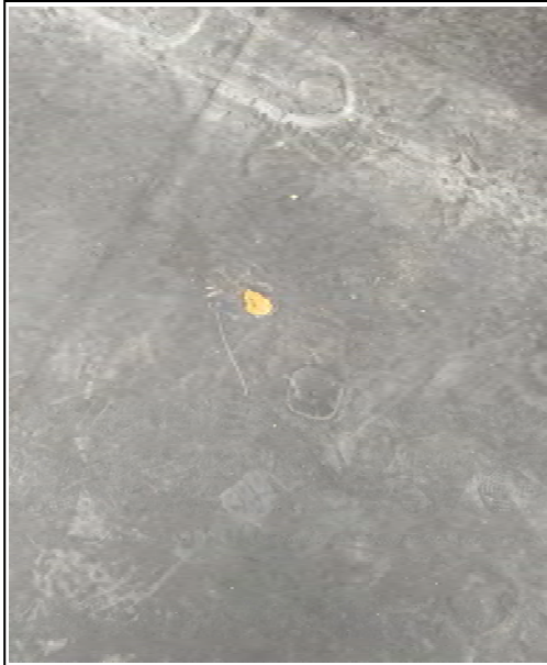
Photograph No. 41 – Lower level roof sampled
