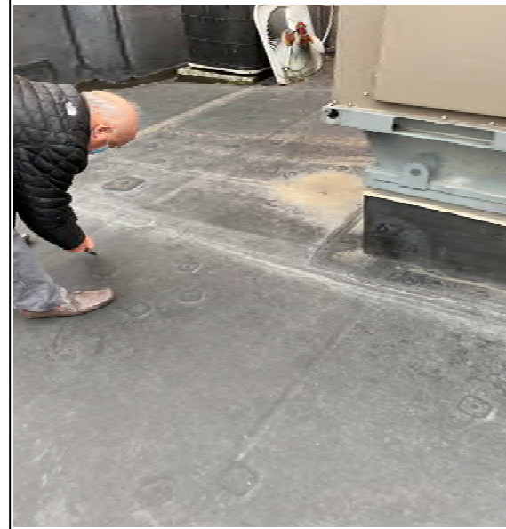
Photograph No. 42 – Lower level roof sampled
