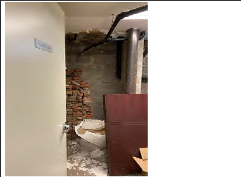
Photograph No. 17– Basement ceiling
