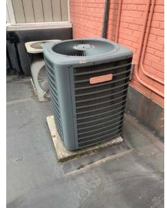
Figure 1: Split System #1 Furnace - Basement Floor Figure 2: Split System #1 Air Condensing Unit - Annex Roof
