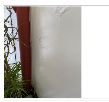
Photograph No. 26 – Damaged wall plaster and paint
