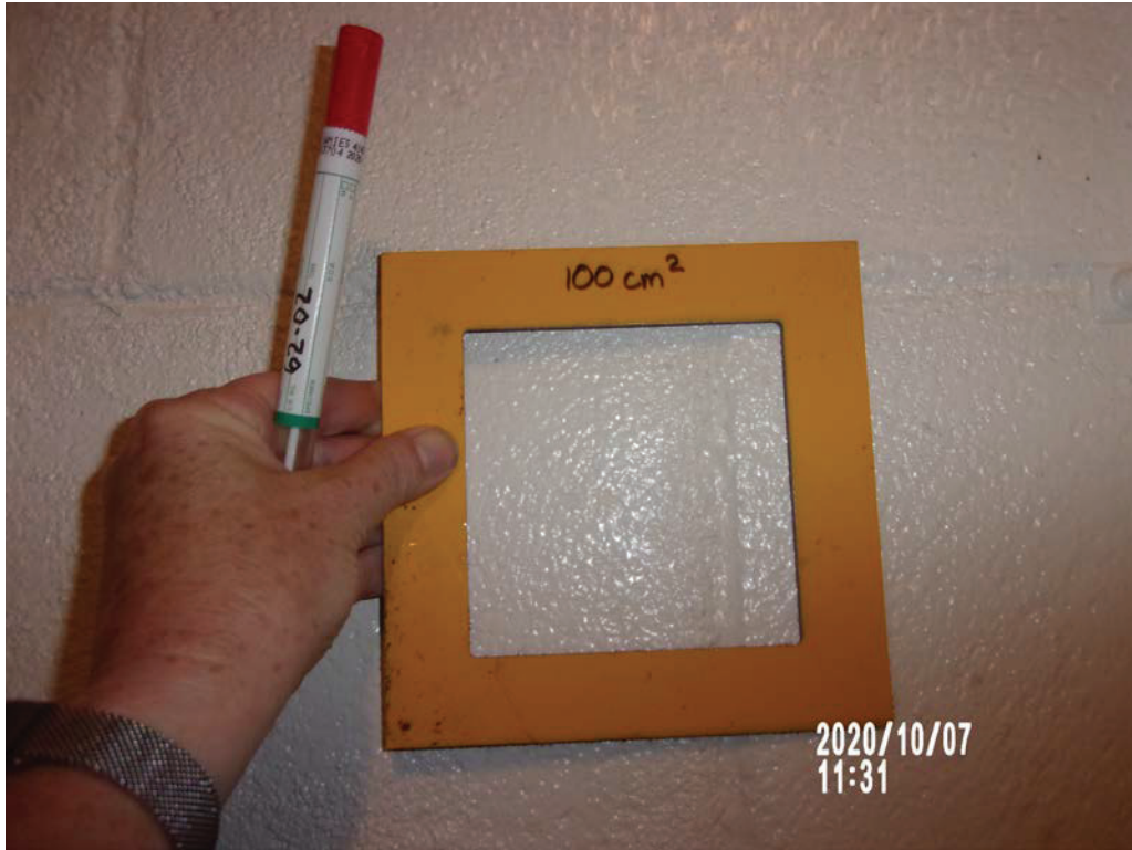
Photo #23 – Swab sample #62-02, Unit #1262 laundry room
