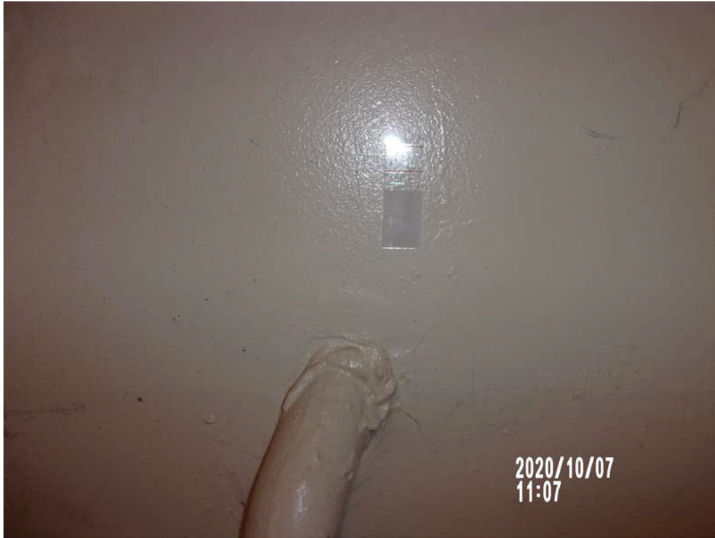
Photo #9 – Tape-lift sample #68-02, Unit #1268 laundry room
