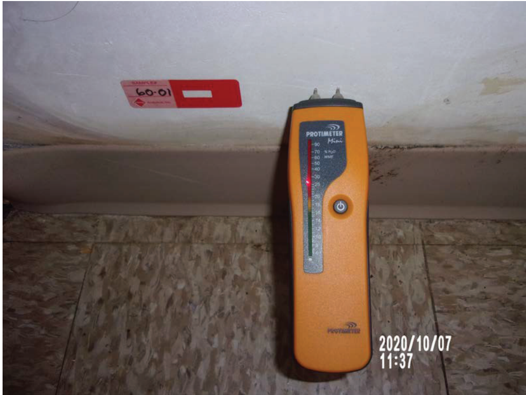
Photo #25 – Moisture meter at red level reading, Unit #1260 living room
