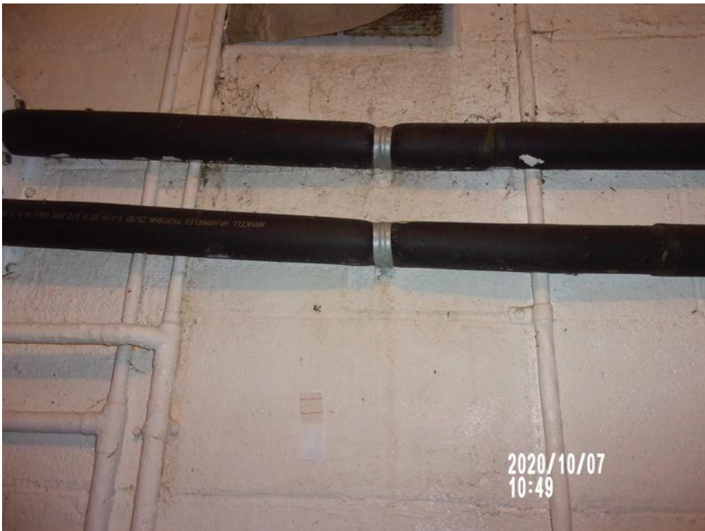
Photo #6 – Tape-lift sample #70-01, Unit #1270 laundry room
