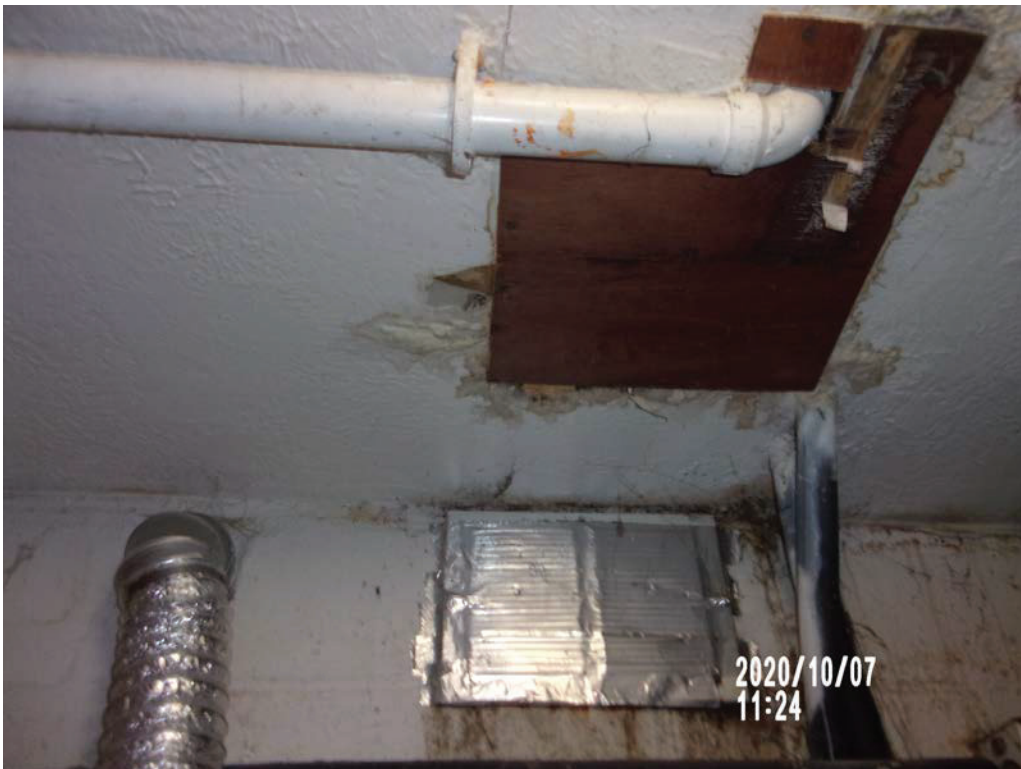
Photo #18 – Bulk sample #64-03, Unit #1264 laundry room
