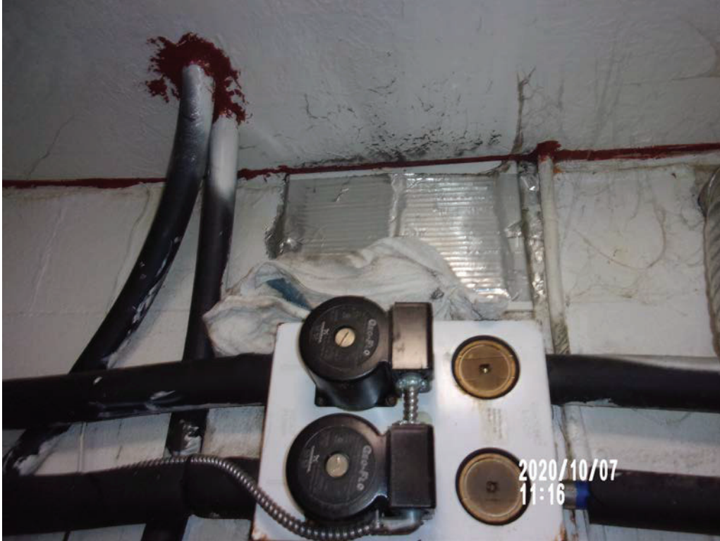
Photo #13 – Unit #1266 laundry room
