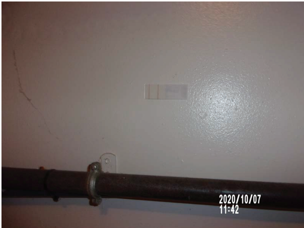
Photo #28 – Tape-lift sample #60-02, Unit #1260 laundry room
