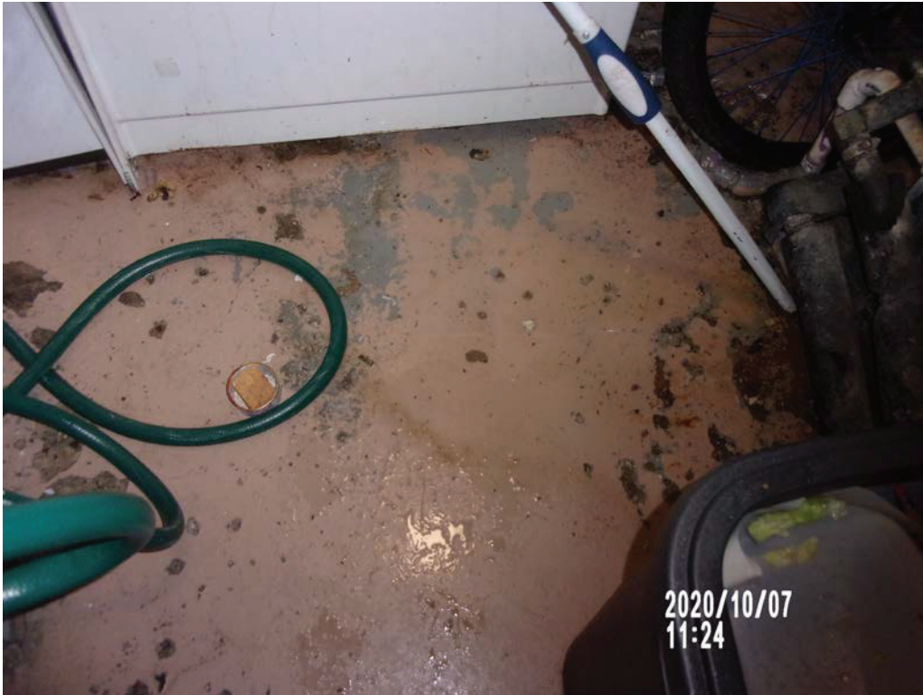
Photo #17 – Unit #1264 laundry room floor
