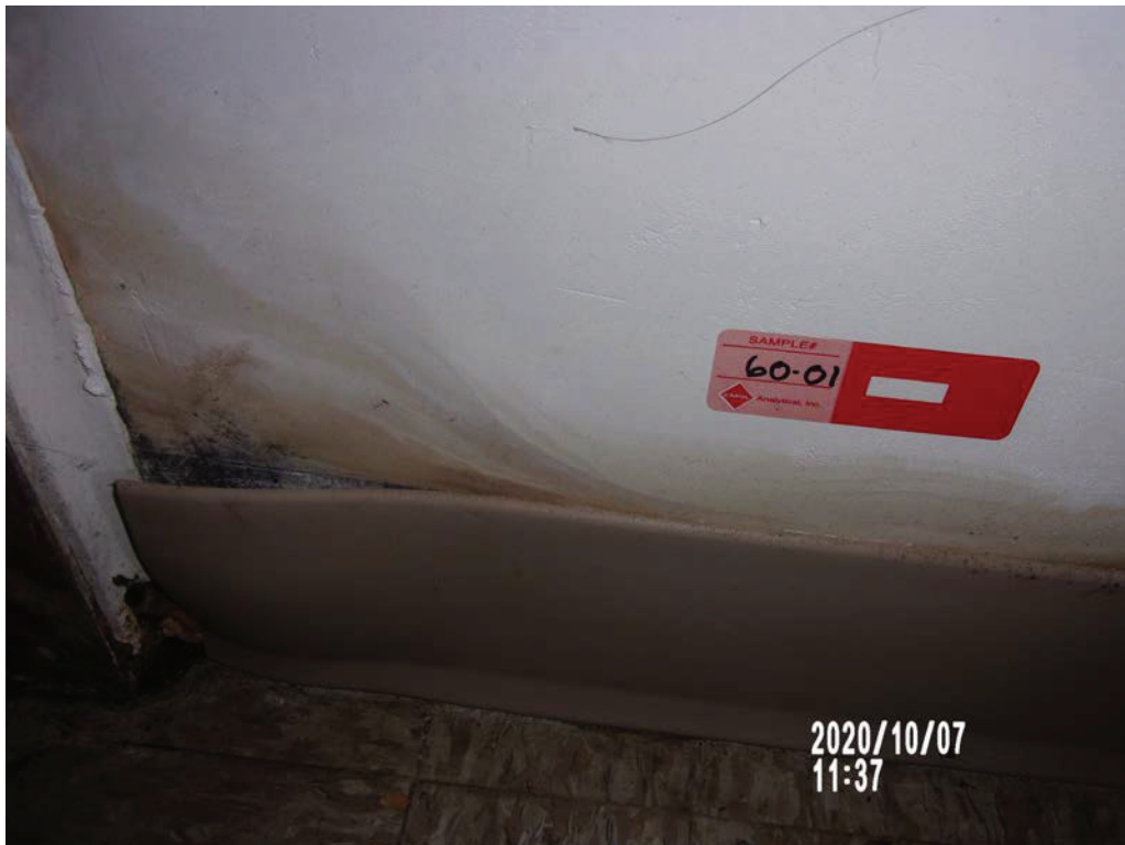
Photo #26 – Tape-lift sample #60-01, Unit #1260 living room
