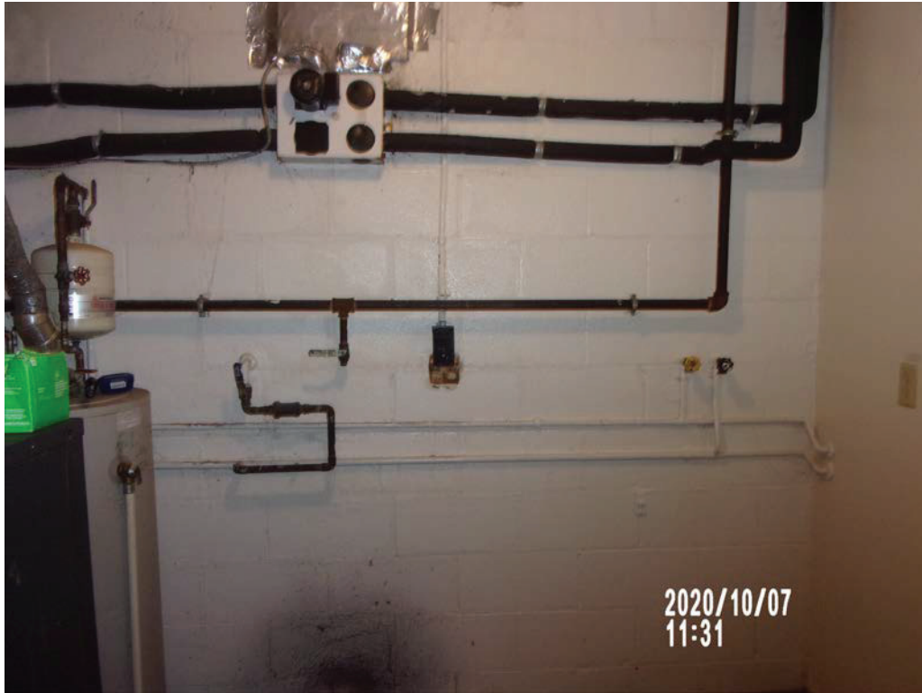
Photo #21 –Unit #1262 laundry room
