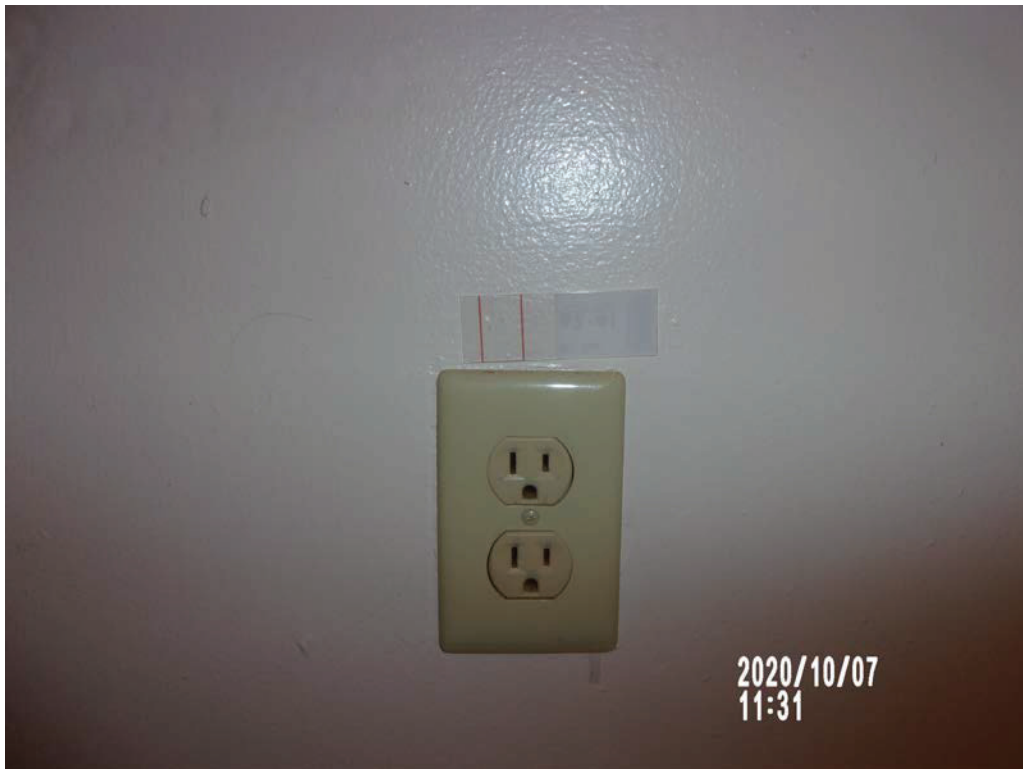
Photo #22 – Tape-lift sample #62-01, Unit #1262 laundry room
