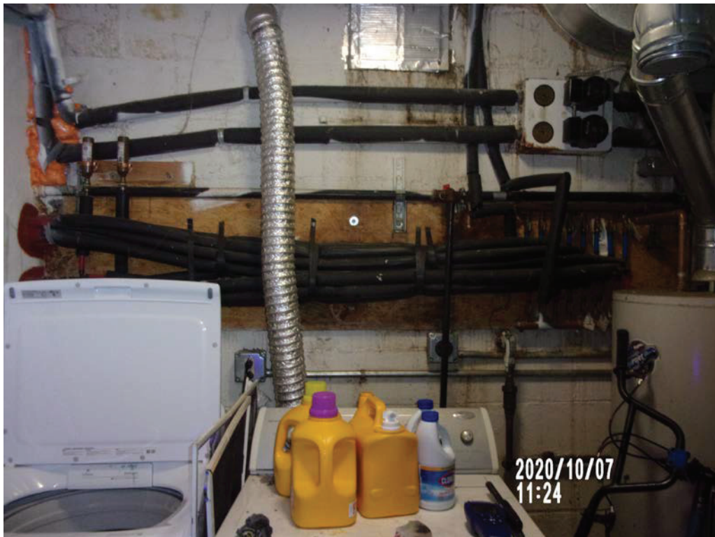
Photo #16 – Unit #1264 laundry room
