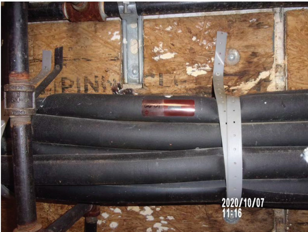
Photo #14 – Tape-lift sample #66-01, Unit #1266 laundry room
