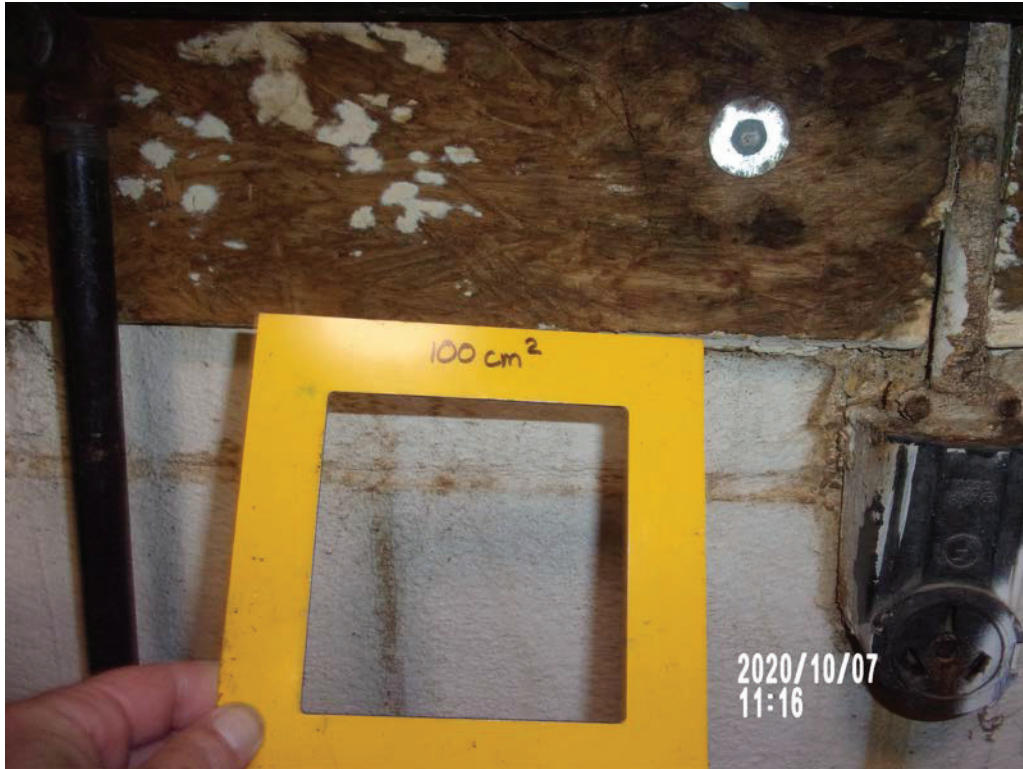
Photo #15 – Swab sample #66-02, Unit #1266 laundry room
