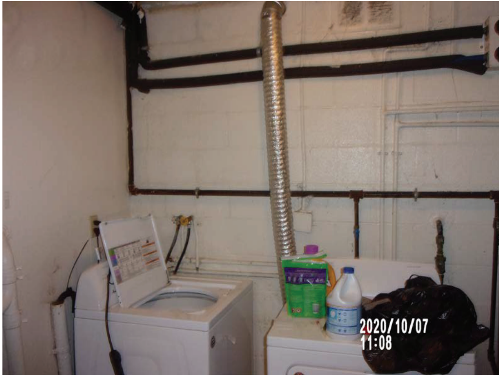
Photo #11 – Unit #1268 laundry room
