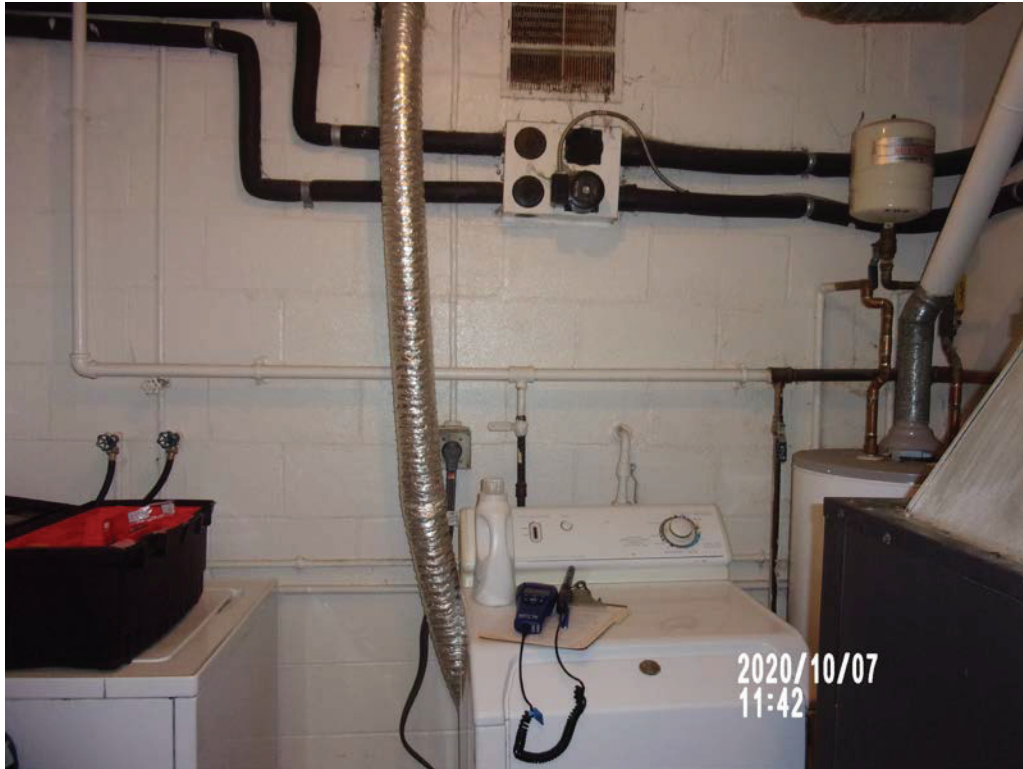
Photo #27 – Unit #1260 laundry room
