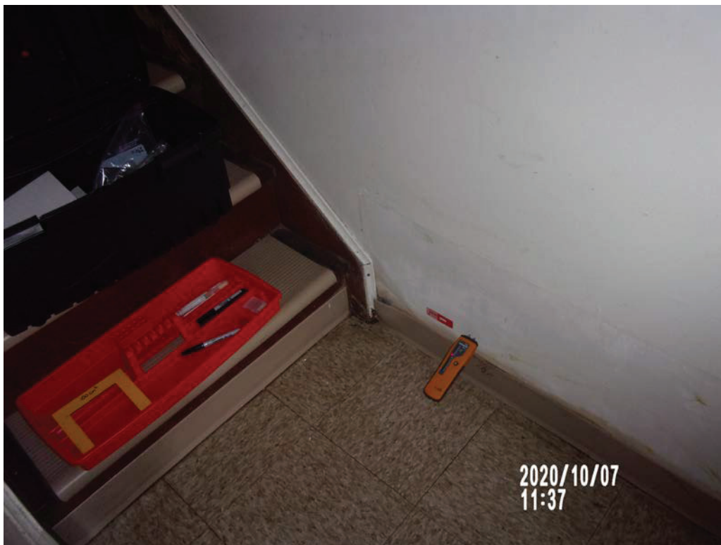
Photo #24 – Damp area by stairway in living room, Unit #1260
