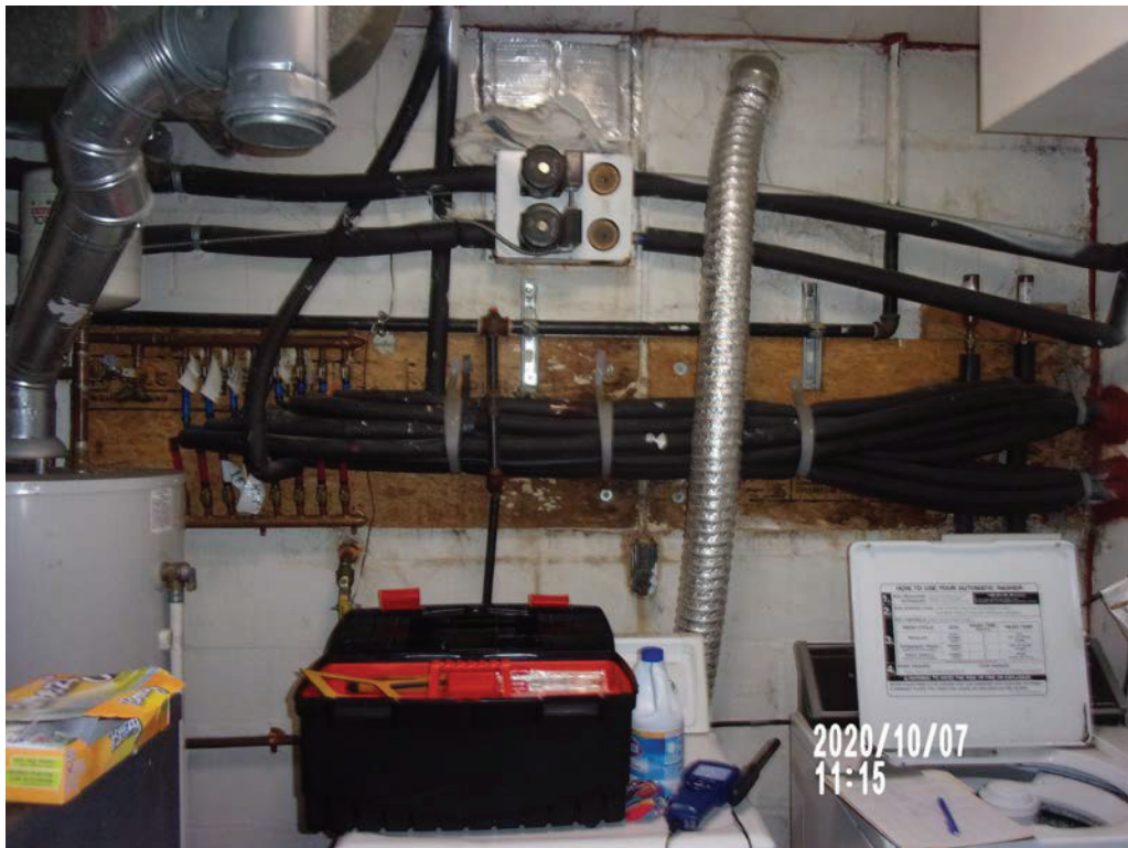
Photo #12 – Unit #1266 laundry room
