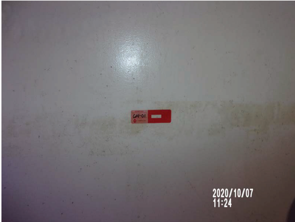
Photo #19 – Tape-lift sample #64-01, Unit #1264 laundry room
