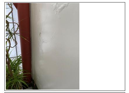
Photograph No. 26 – Damaged wall plaster and paint
