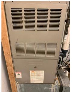
Goodman Unknown GSC130603CB Direct Vent Natural Gas Furnace and Condensing Unit 1 13.0 Seasonal Energy Efficiency Ratio (SEER) or 11.0 Energy Efficiency Ratio (EER) 80% Annual Fuel Utilization Efficiency (AFUE) 1 Heating, 1 Cooling R-22 Unknown (~80.0 MBH) – Heating 5 Tons, 60.0 MBH - Cooling None
