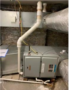
Goodman (condensing unit) & Ducane (furnace) Unknown CK60-3C Direct Vent Natural Gas Furnace and Condensing Unit 1 13.0 Seasonal Energy Efficiency Ratio (SEER) 80% Annual Fuel Utilization Efficiency (AFUE) 1 Heating, 1 Cooling R-22 Unknown (~80.0 MBH) – Heating 5 Tons, 60.0 MBH - Cooling None
