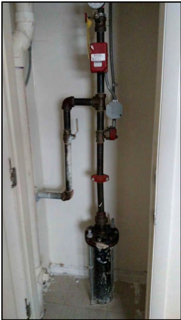
TYPICAL SPRINKLER RISER WITH DEVICES 6
