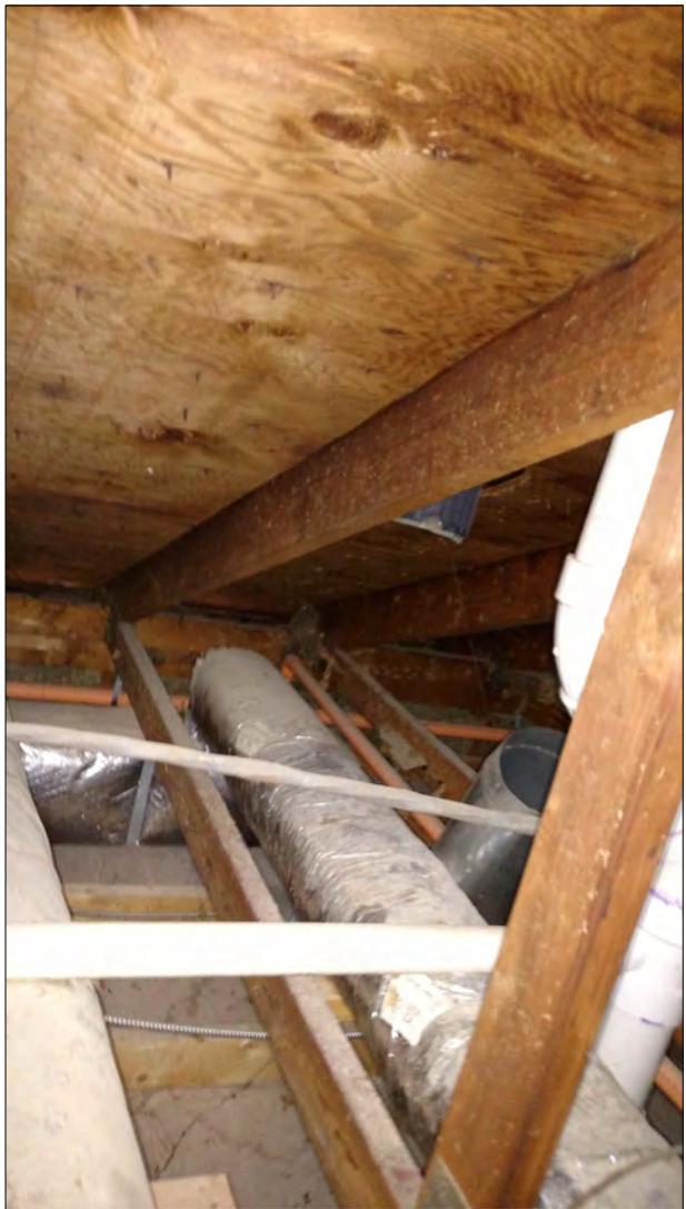
1332 HEART LOCATION SPRINKLER PIPING NO INSULATION IN ATTIC 13
