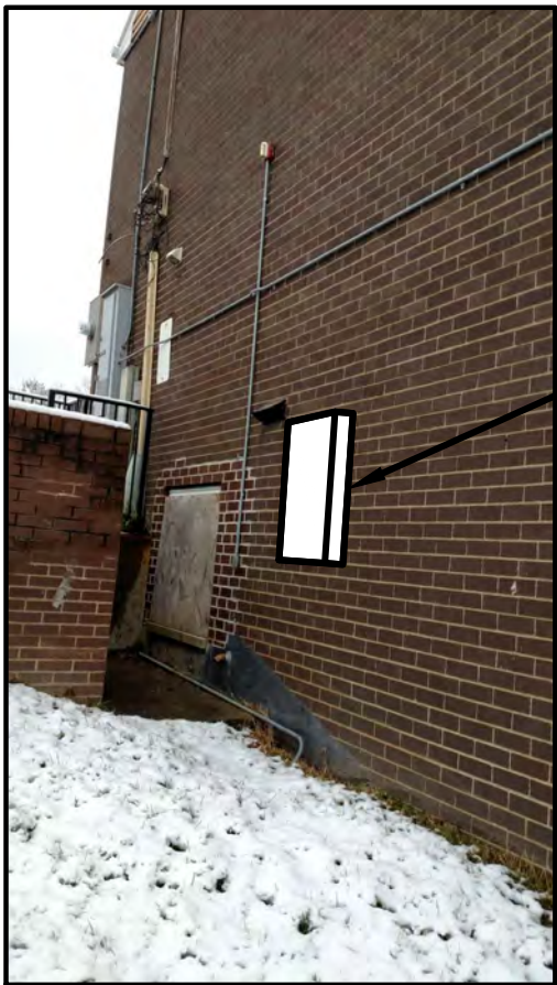
NOLAN LOCATION FOR RELOCATED EXTERIOR FA PANEL 5
