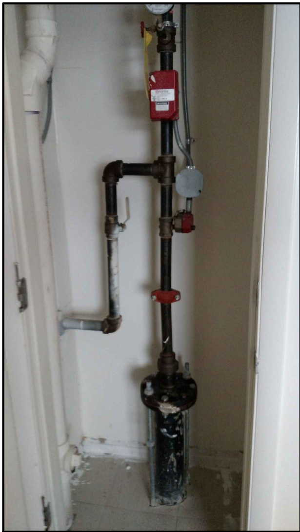
TYPICAL SPRINKLER RISER WITH DEVICES 6 SCALE: NONE
