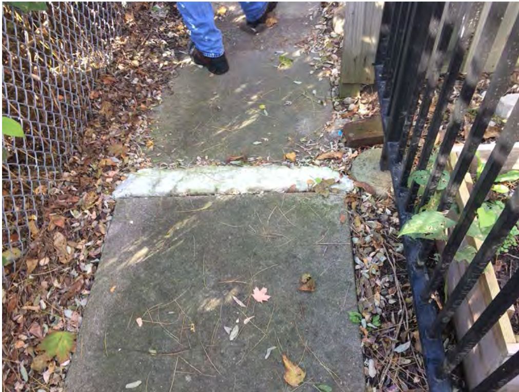
Photo 105 – Replace 3'x4' slab [Plan Sheet SP-9]
