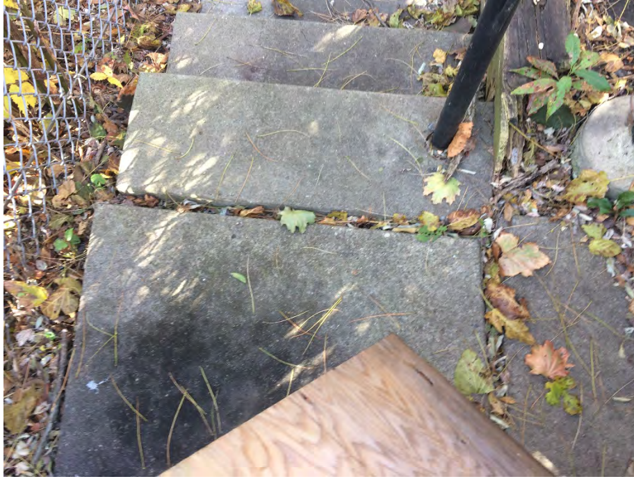
Photo 104 – Clean, neoprene, and caulk joint [Plan Sheet SP-9]
