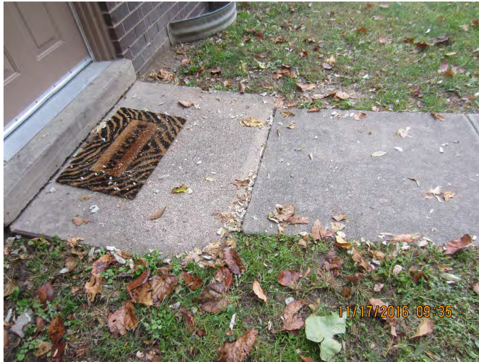
Photo 59 –Foam lift slab [Plan Sheet SP-4]
