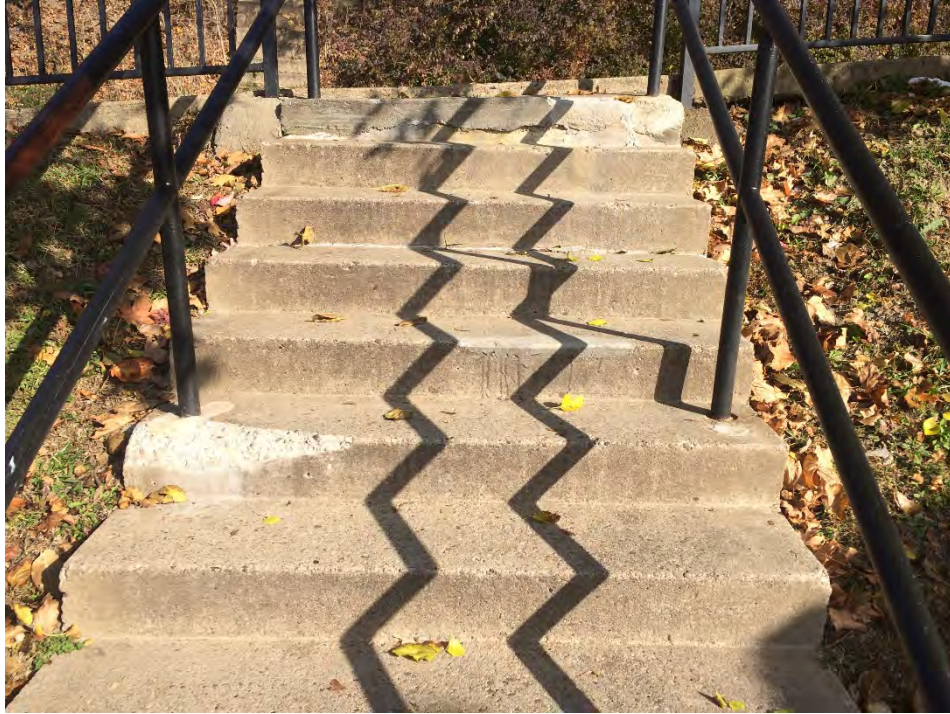
Photo 96 – Replace 2 concrete steps [Plan Sheet SP-9]
