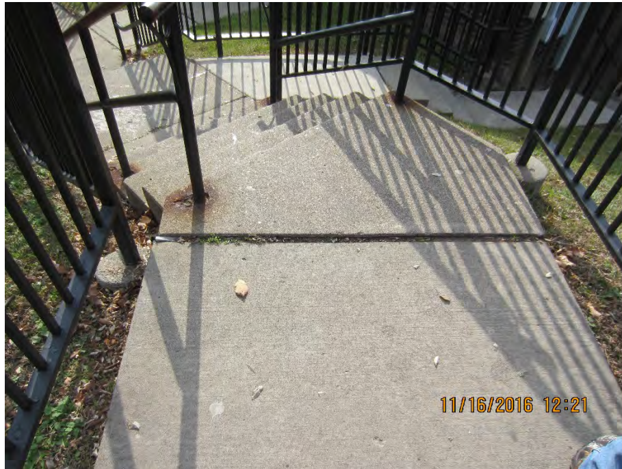
Photo 11 – Grind & caulk 6' slab [Plan Sheet SP-2]
