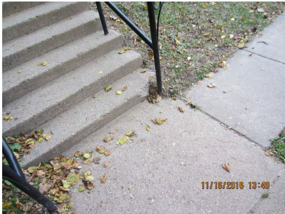
Photo 88 – Repair spalled concrete on steps [Plan Sheet SP-7]
