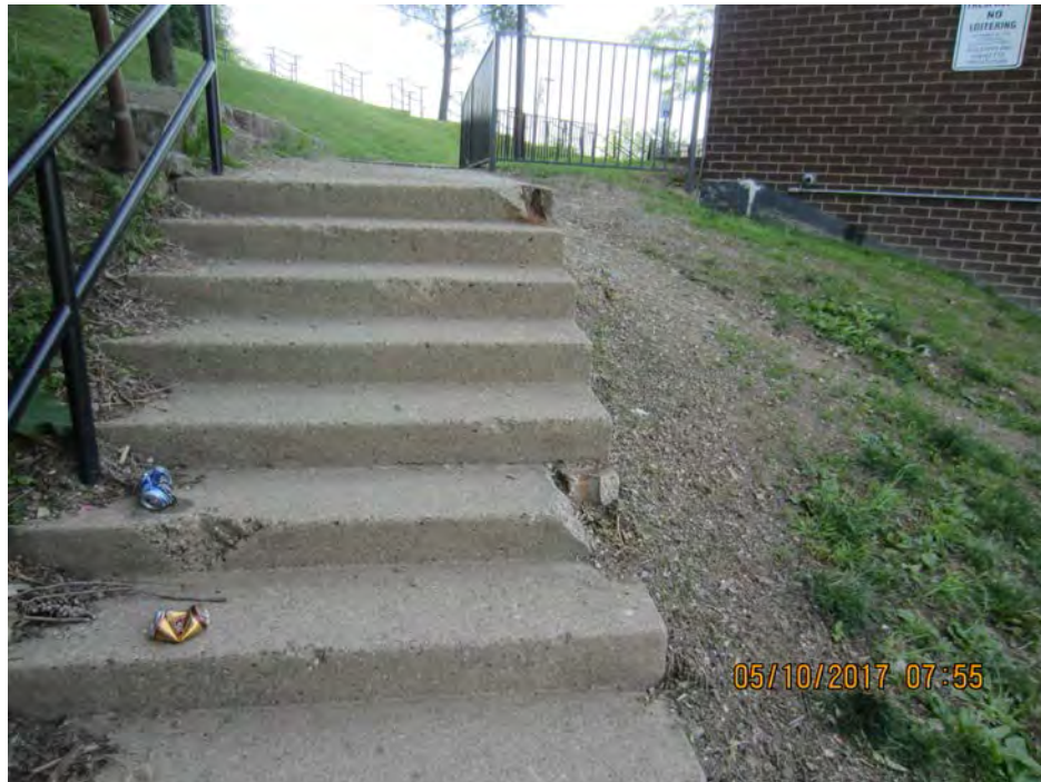
Photo 87 – Repair spalled concrete on steps. Install new section of fence between end of existing fence and handrail. [Plan Sheet SP-7]
