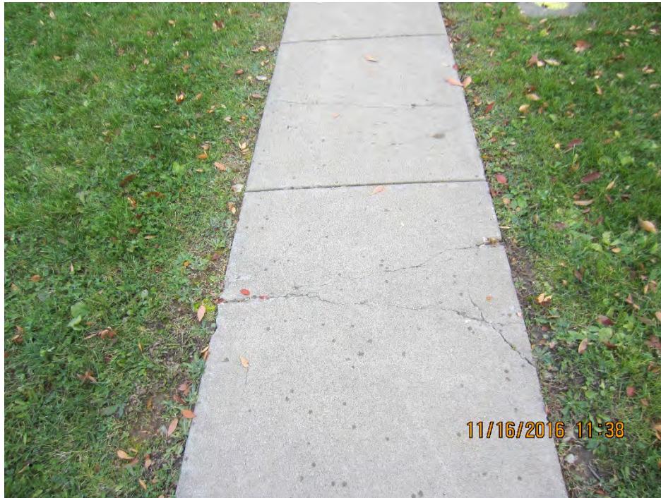
Photo 7 – Crack seal & caulk 3 cracks [Plan Sheet SP-1]
