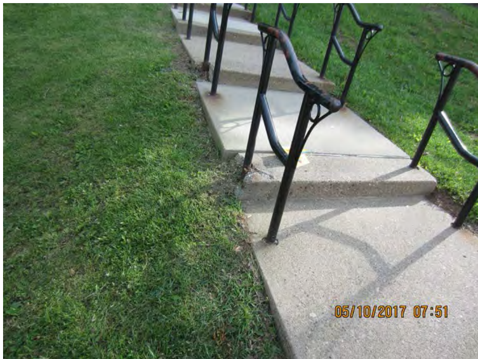
Photo 89a – Repair spalled concrete on steps [Plan Sheet SP-7]
