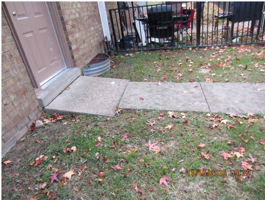
Photo 25 – Foam lift slab [Plan Sheet SP-3]
