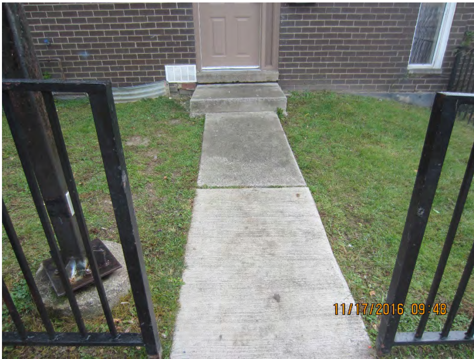
Photo 46 –Foam lift slab. Topsoil and seed area. [Plan Sheet SP-3]
