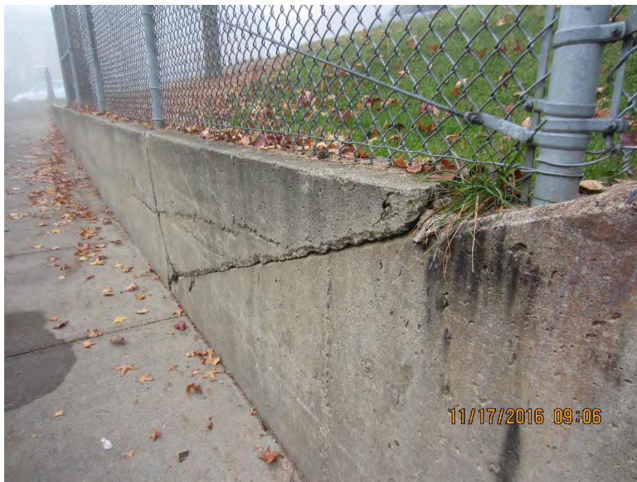
Photo 29 – Repair concrete wall [Plan Sheet SP-3]
