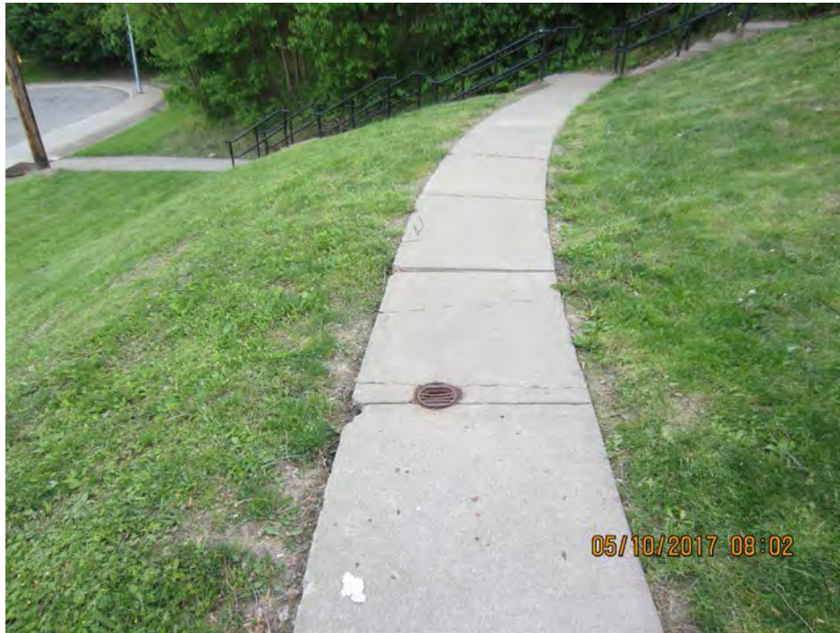
Photo 89f – Replace concrete slab and sewer vent. [Plan Sheet SP-7]
