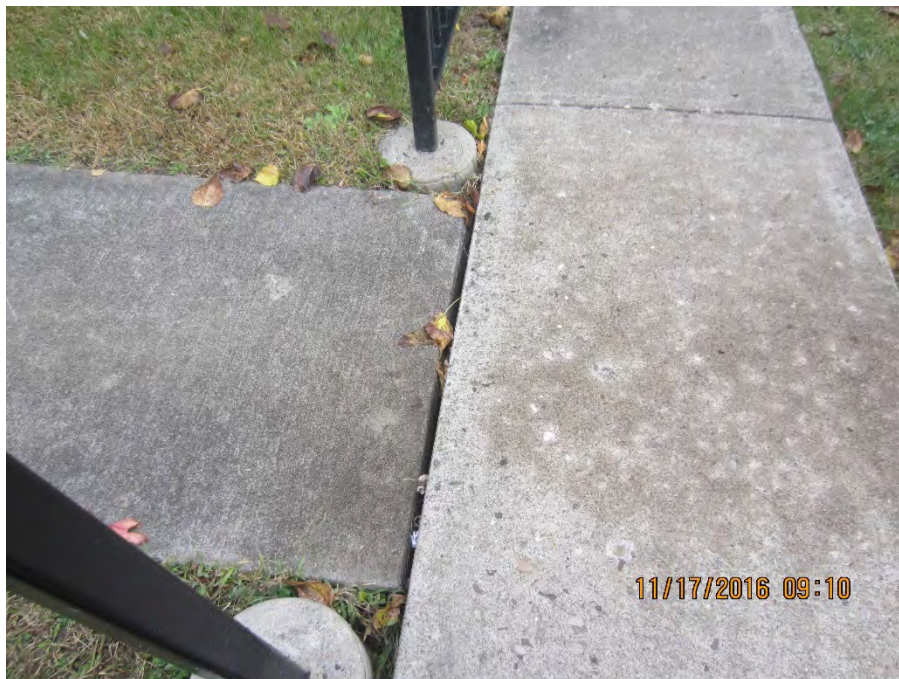
Photo 33 – Neoprene pad joint fill [Plan Sheet SP-3]
