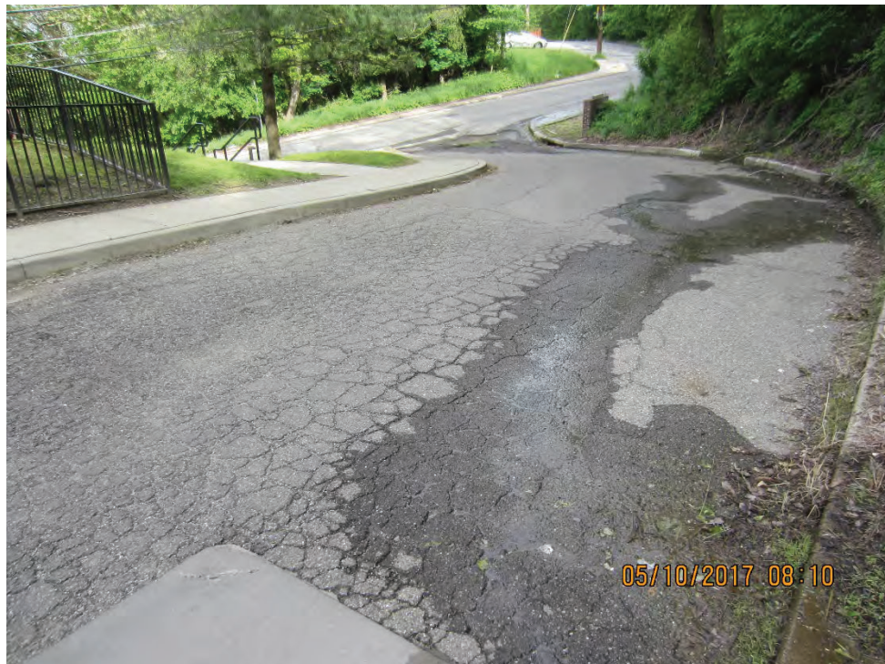
Photo 6b – Drainage issues along the driveway
