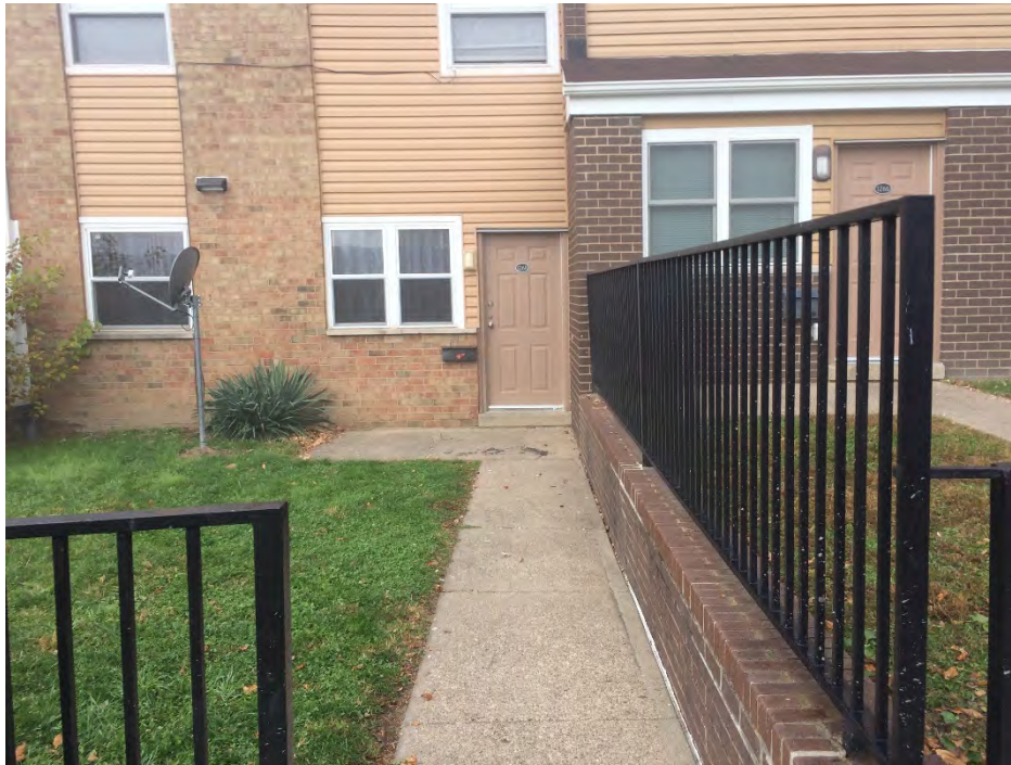
Photo 67 – Neoprene pad crack fill between sidewalk and brick wall [Plan Sheet SP-5]
