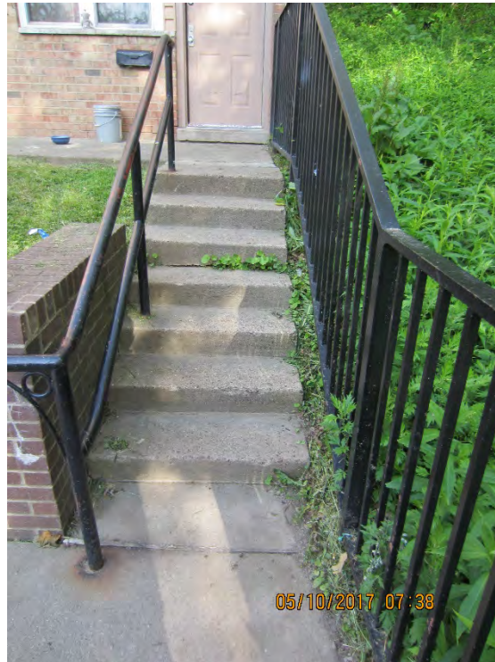
Photo 57 –Topsoil and seed area around landing. Clean debris, grout and caulk step separation.
