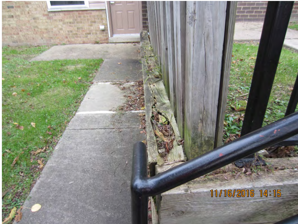
Photo 94 – Foam lift and caulk slab. [Plan Sheet SP-8]
