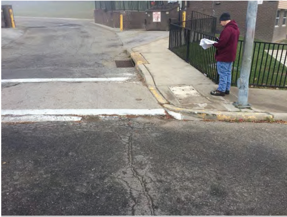
Photo 18A – ADA Truncated Dome to be Replaced
