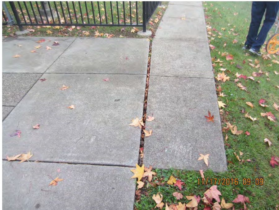
Photo 32 – Neoprene pad joint fill [Plan Sheet SP-3]
