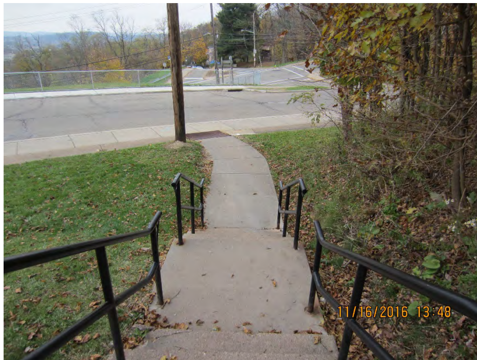
Photo 84 – Repair spalled concrete on steps [Plan Sheet SP-7]
