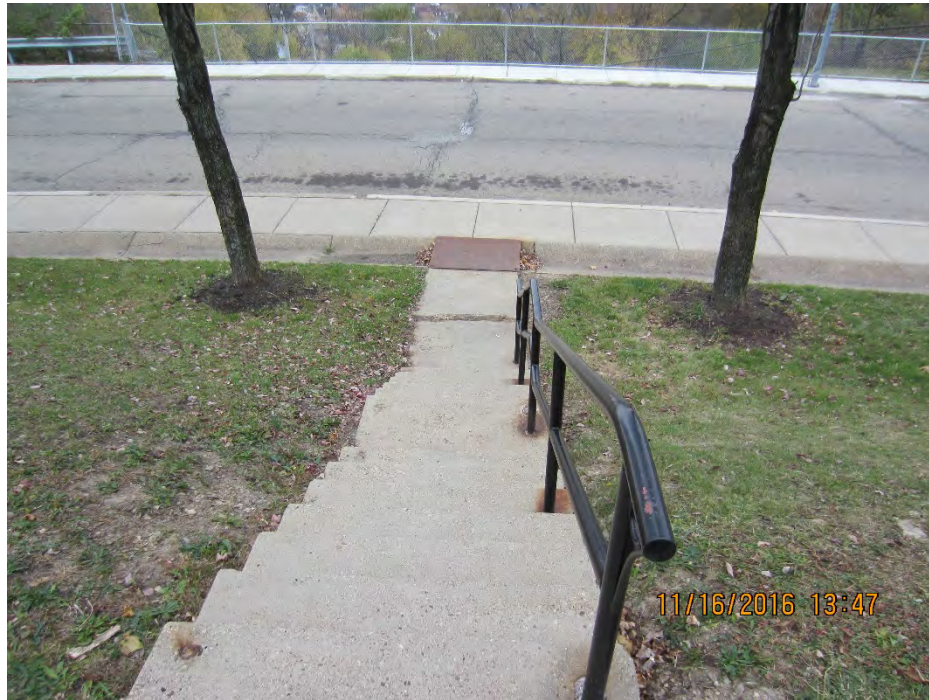
Photo 83 – Sawcut and install new 4'x6' concrete slab [Plan Sheet SP-7]
