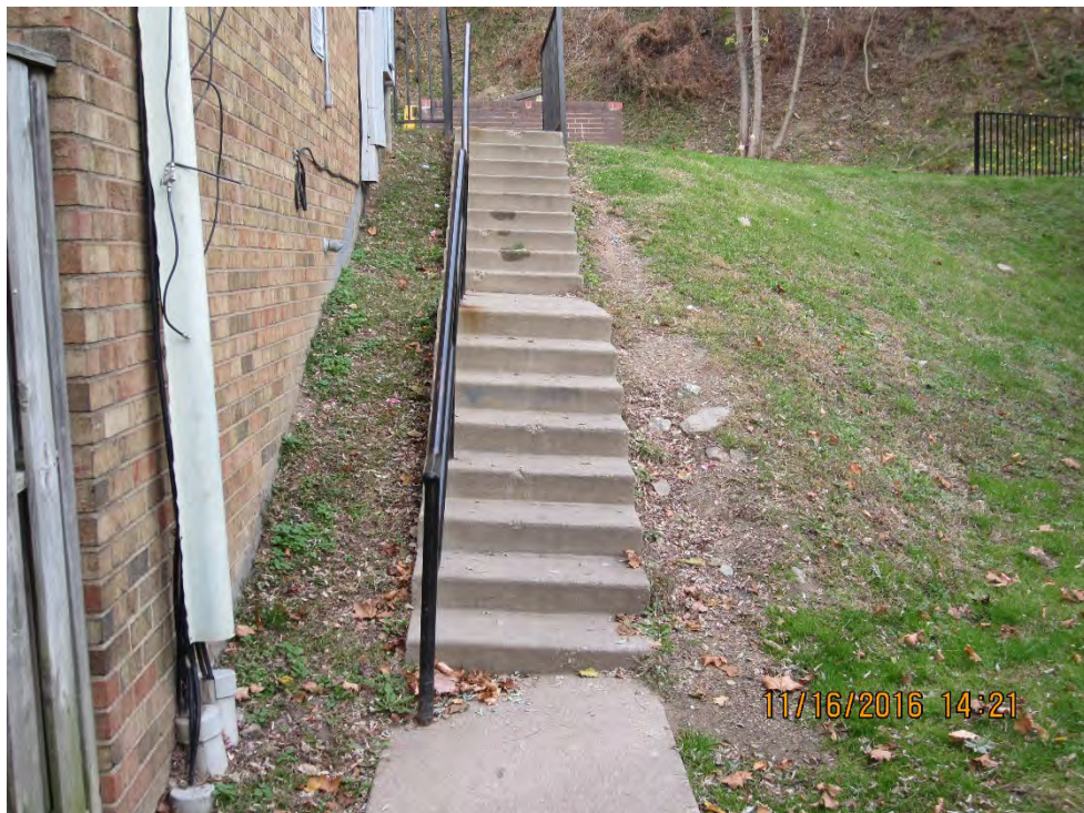
Photo 91 – Foam lift concrete staircase [Plan Sheet SP-8]
