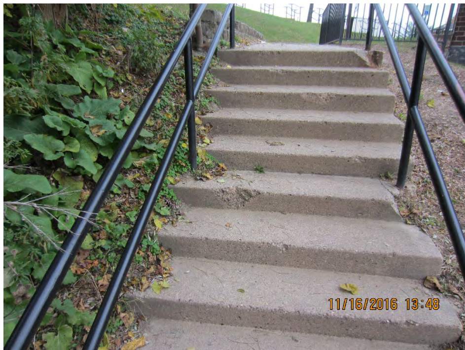
Photo 86 – Repair spalled concrete on steps [Plan Sheet SP-7]
