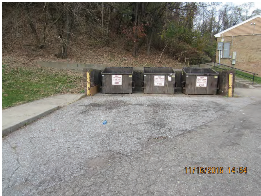
Photo 9 – Concrete area to be removed and replaced with asphalt.
