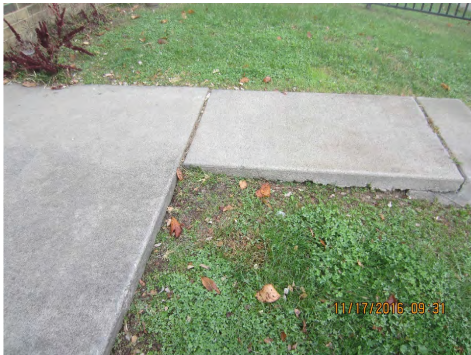
Photo 52 –Foam lift slab [Plan Sheet SP-4]
