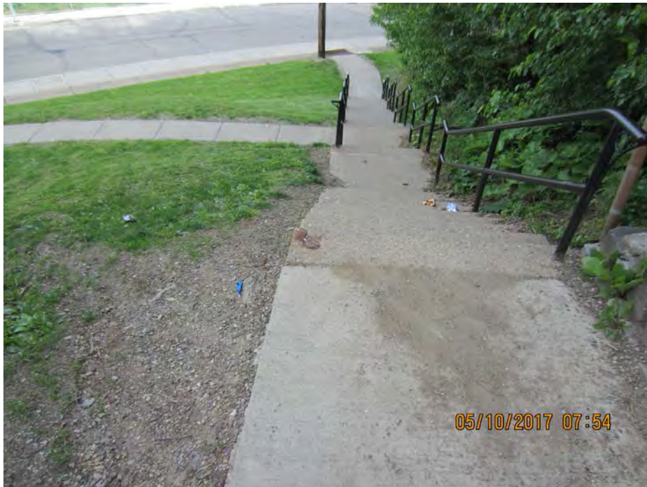
Photo 89c – Replace missing handrail. Topsoil and seed area. [Plan Sheet SP-7]
