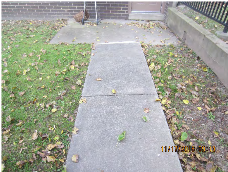
Photo 37 – Replace completely heaved sidewalk [Plan Sheet SP-3]
