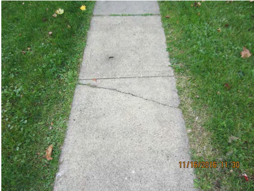
Photo 8a – Clean crack & joint seal [Plan Sheet SP-2]
