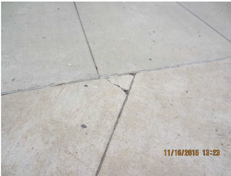
Photo 76 – Clean and caulk crack [Plan Sheet SP-6]
