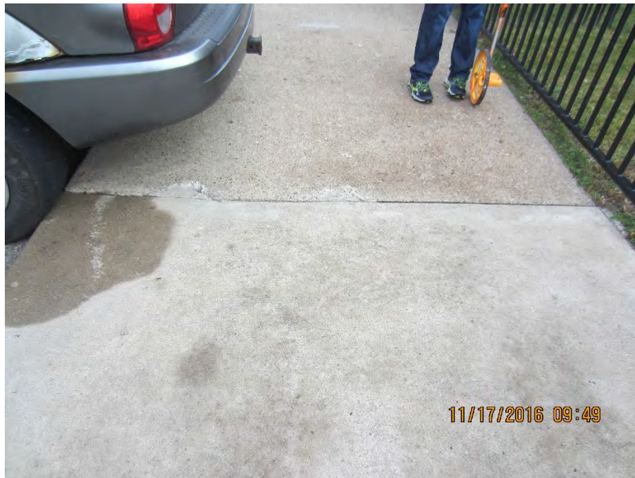
Photo 68b –Clean and joint seal cracks [Plan Sheet SP-3]
