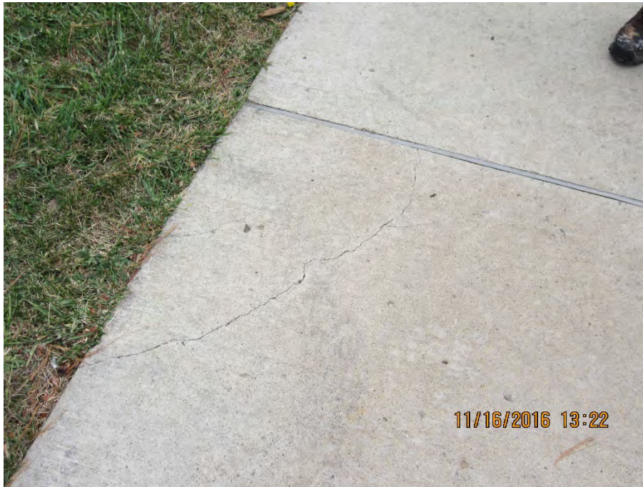
Photo 75 – Clean and caulk crack [Plan Sheet SP-6]
