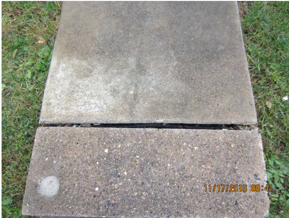
Photo 49 – Neoprene joint fill [Plan Sheet SP-3]
