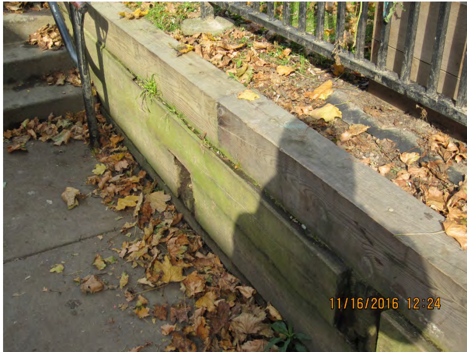
Photo 12 – Remove & replace 3' high railroad tie wall [Plan Sheet SP-2]
