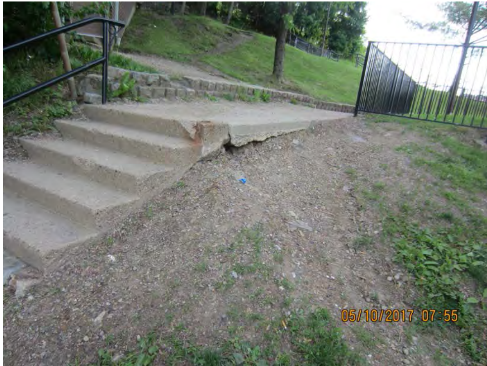
Photo 89d – Foam level slab and backfill and seed area. [Plan Sheet SP-7]
