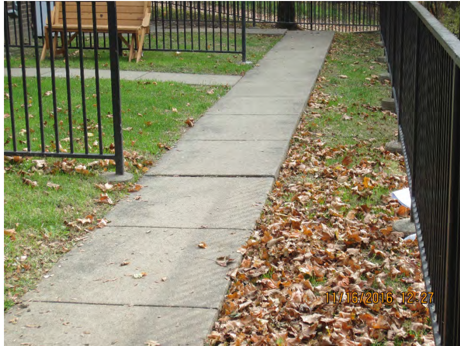
Photo 15 – Grind & caulk 3' slab [Plan Sheet SP-2]
