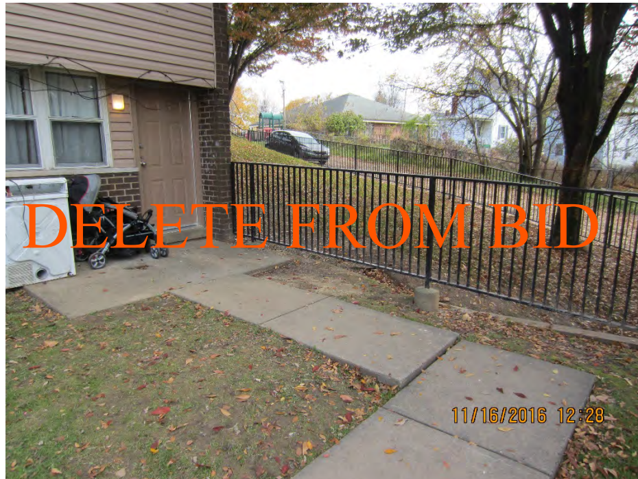
Photo 16 – Foam lift slab, grind & caulk 3' slab [Plan Sheet SP-2]
