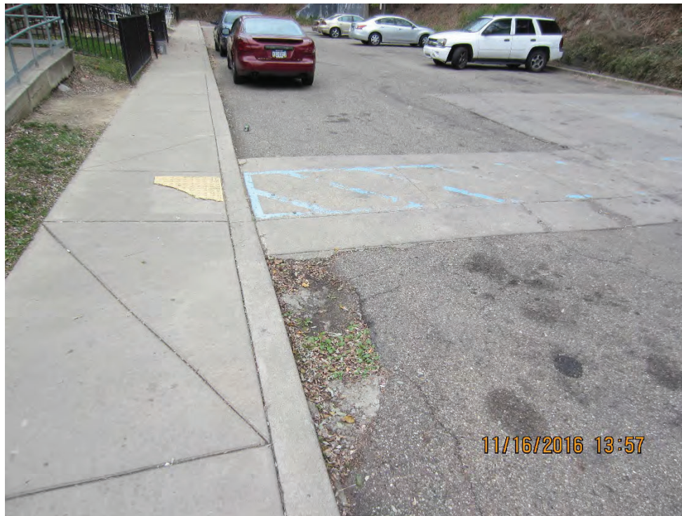
Photo 6a – Remove and replace truncated domes
