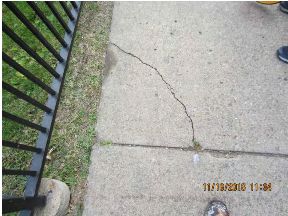
Photo 8b – Clean crack & joint seal [Plan Sheet SP-2]
