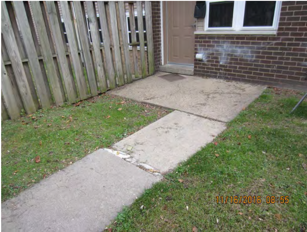
Photo 95c – Grind slab Sheet SP-8]
