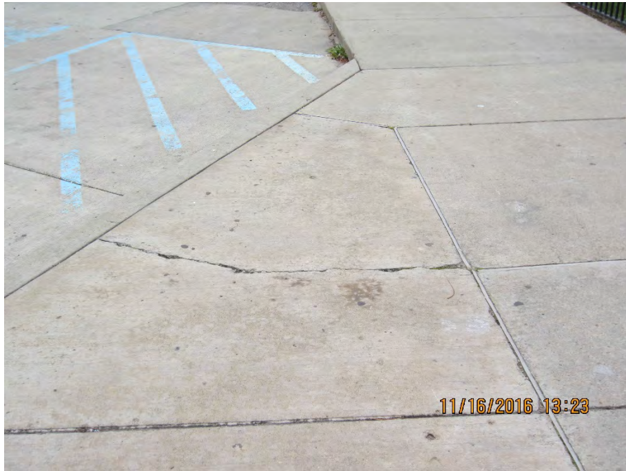
Photo 77 – Clean and caulk crack [Plan Sheet SP-6]
