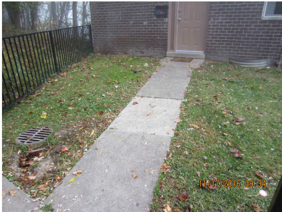
Photo 58 –Foam lift slab. Topsoil and seed around inlet [Plan Sheet SP-4]
