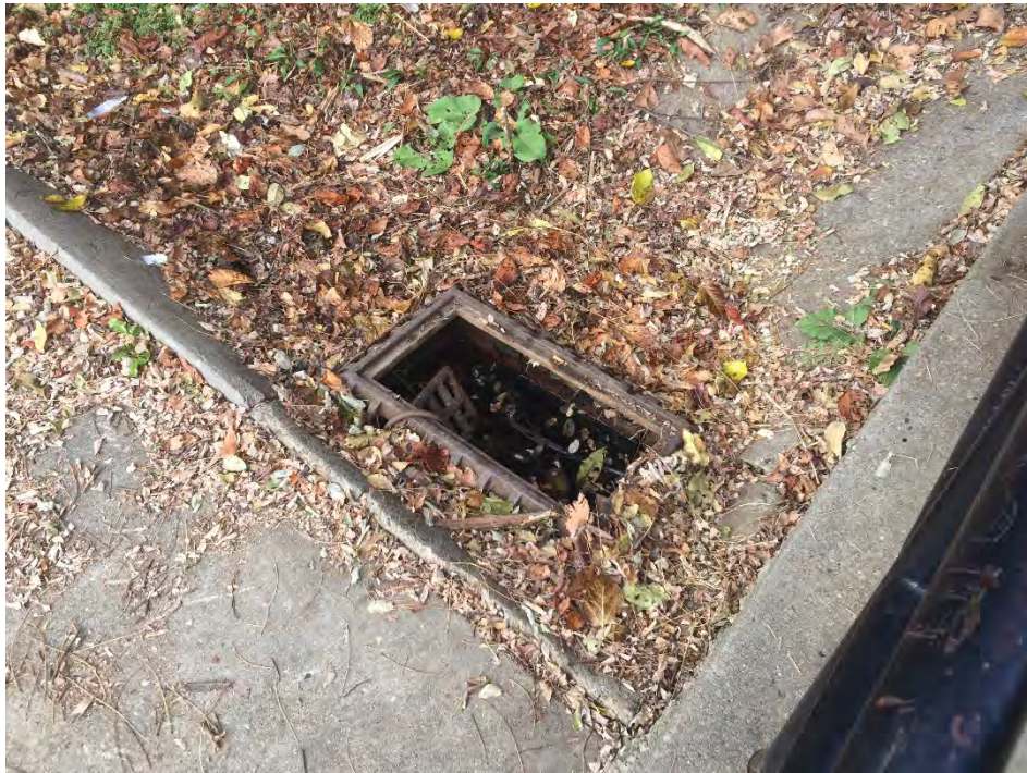
Photo 60 – Clean out and reset inlet grate [Plan Sheet SP-4]
