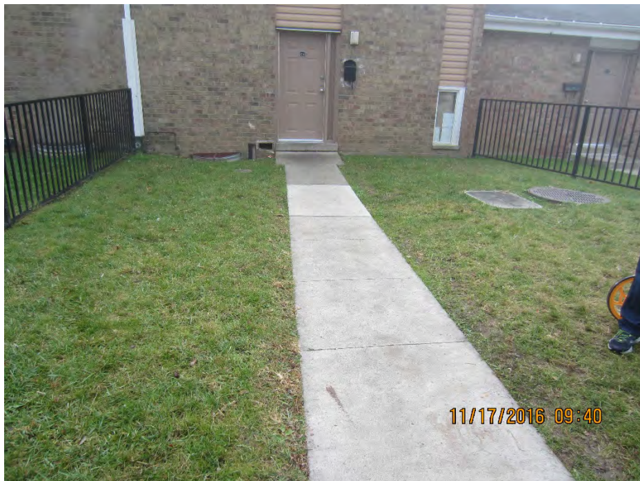
Photo 50 –Foam lift slab [Plan Sheet SP-4]
