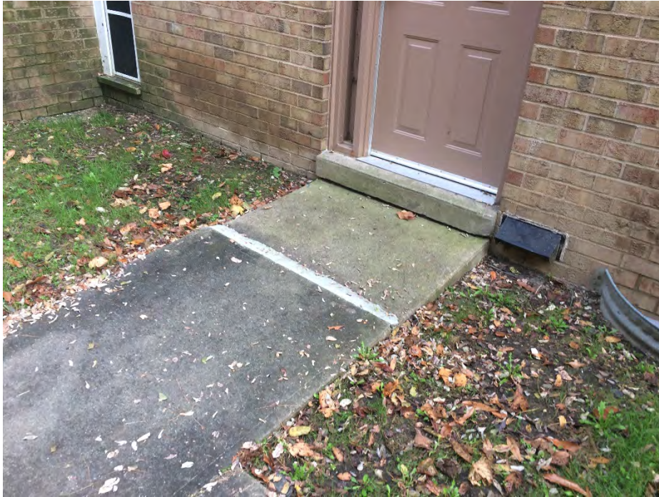
Photo 61 – Foam lift slab [Plan Sheet SP-4]
