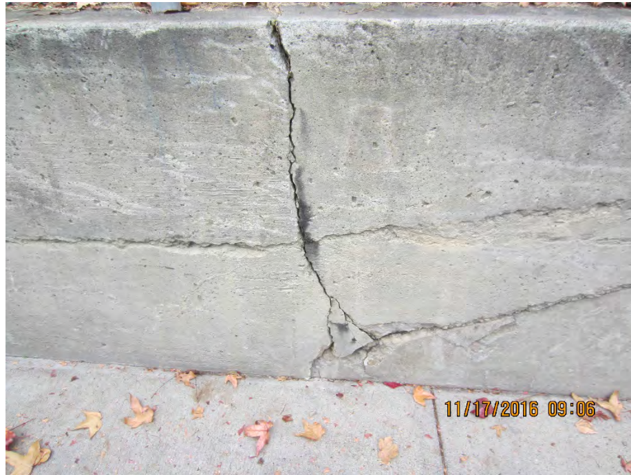
Photo 28 – Repair concrete wall [Plan Sheet SP-3]
