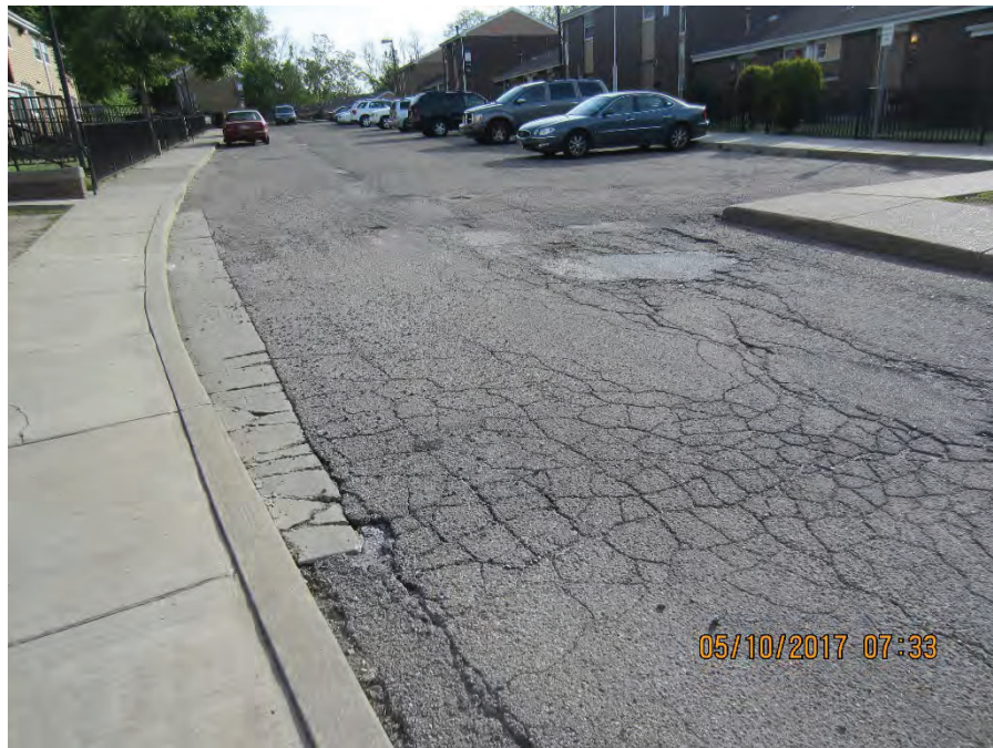
Photo 9 – Concrete area to be removed and replaced with asphalt.
