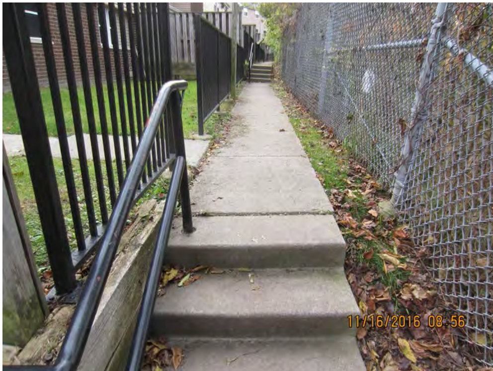
Photo 95b – Grind slab Sheet SP-8]
