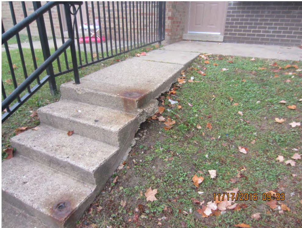
Photo 55 –Backfill and foam lift under steps [Plan Sheet SP-4]
