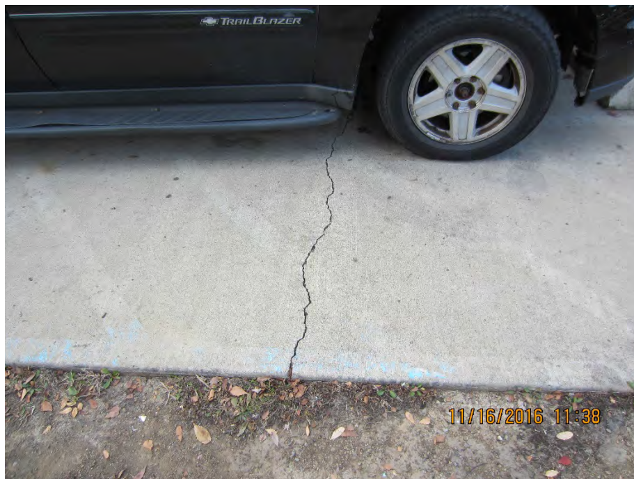
Photo 6 – Crack seal & caulk handicapped parking area [Plan Sheet SP-1]
