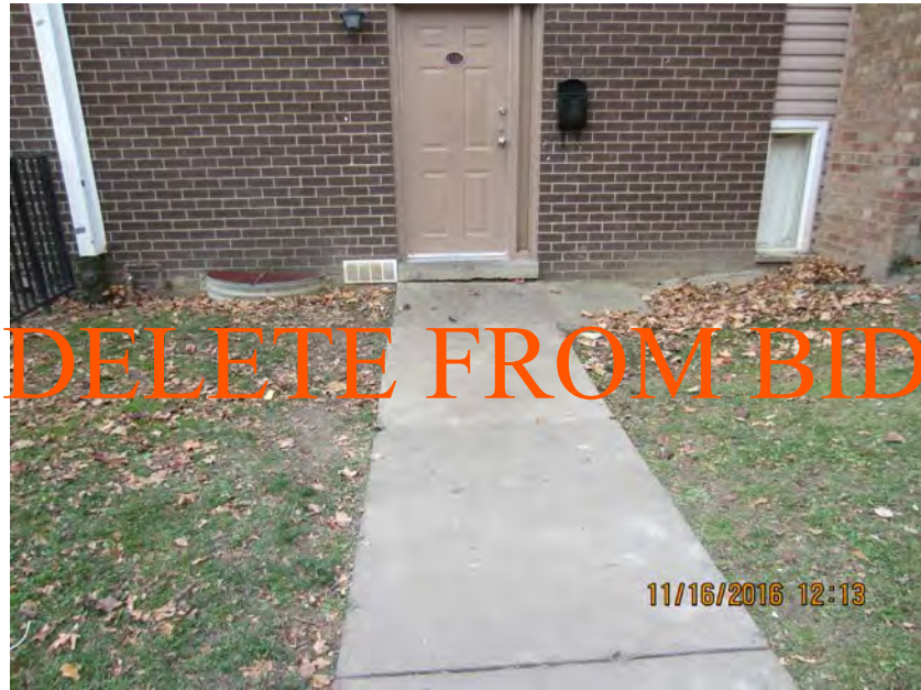
Photo 10c – Foam lift slab [Plan Sheet SP-2]
