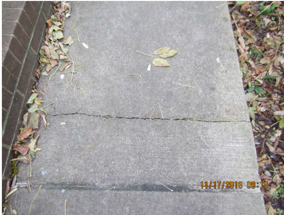
Photo 40 – Clean crack & joint seal [Plan Sheet SP-3]
