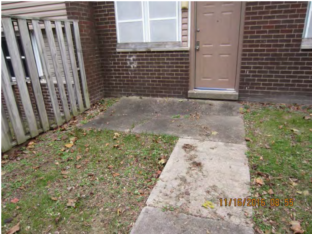
Photo 95a – Replace concrete slab [Plan Sheet SP-8]
