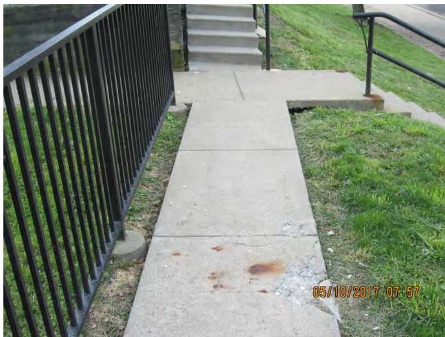
Photo 82a – Replace concrete slab. Foam level slab at top of steps Backfill and seed around slab at top of steps. [Plan Sheet SP-6]
