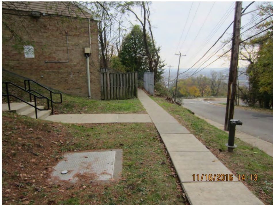
Photo 94 – Foam lift and caulk slab. [Plan Sheet SP-8]
