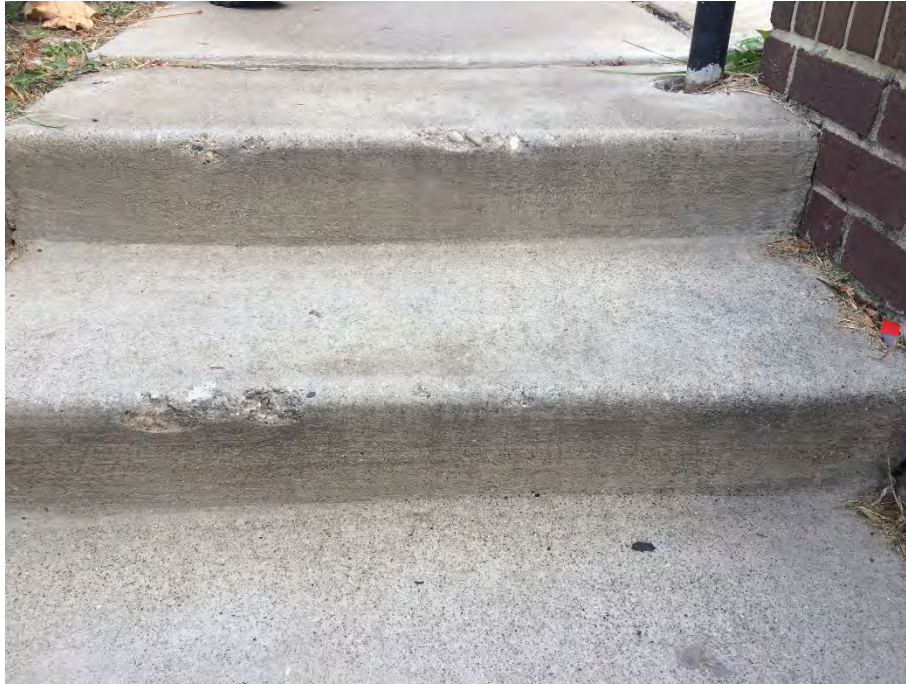
Photo 71 – Grind top of step [Plan Sheet SP-5]
