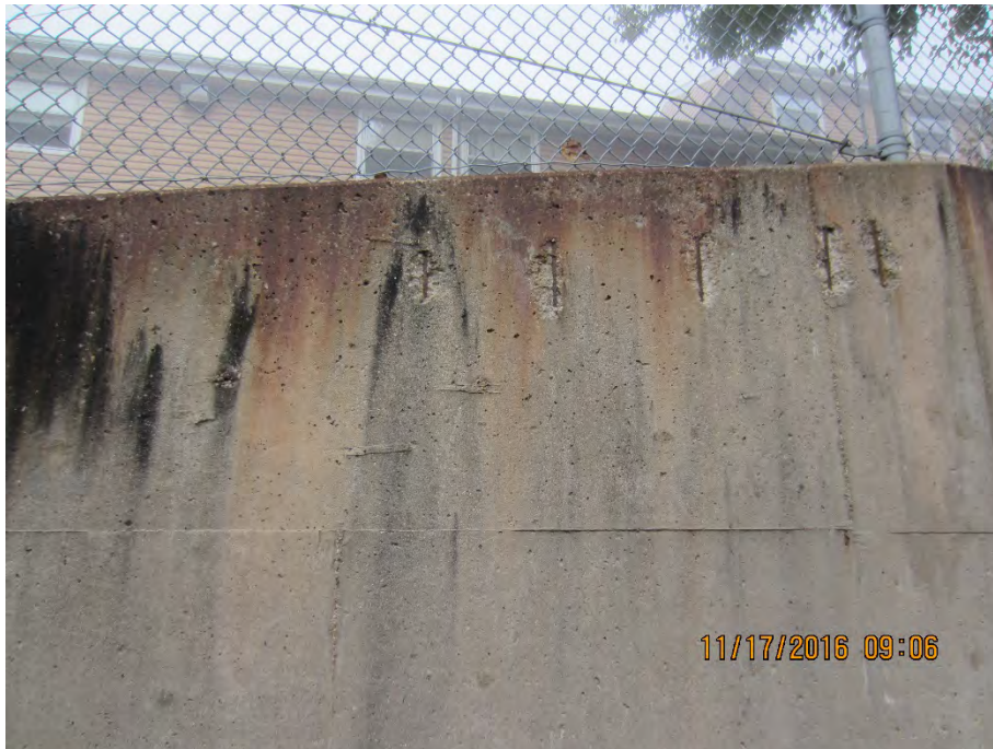
Photo 30 – Repair exposed rebar [Plan Sheet SP-3]
