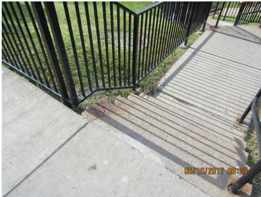
Photo 11a – Replace missing 6.5' handrail [Plan Sheet SP-2]
