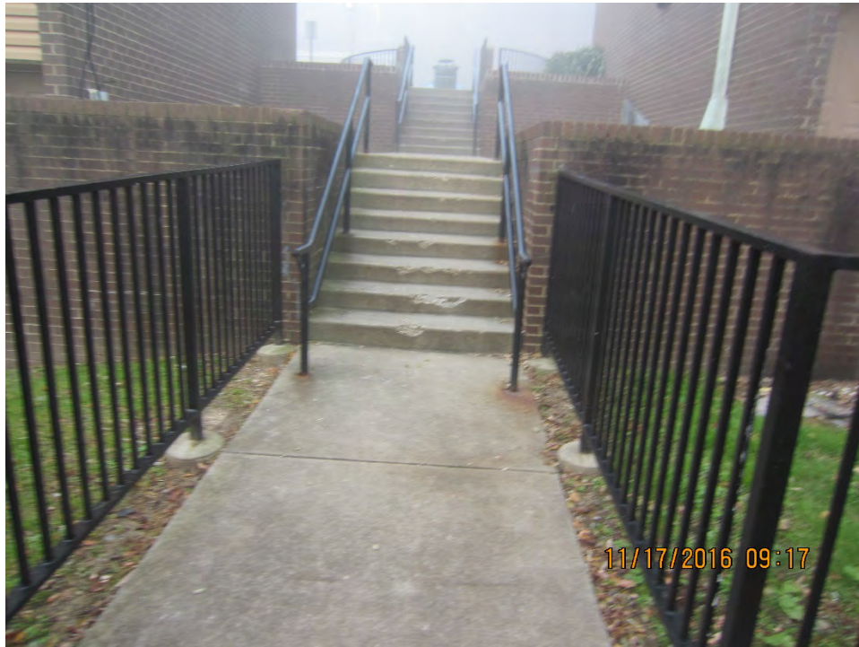
Photo 42 – Repair spalling on concrete staircase [Plan Sheet SP-3]
