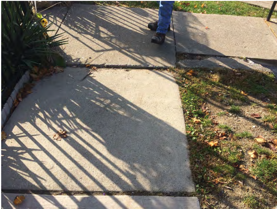
Photo 97 – Foam lift slab [Plan Sheet SP-9]
