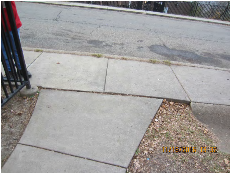
Photo 78 – Grind 5' slab [Plan Sheet SP-6]
