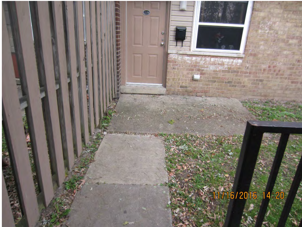
Photo 92 – Foam lift slab [Plan Sheet SP-8]
