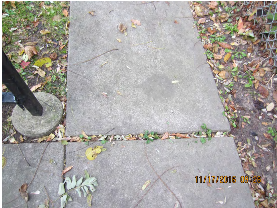
Photo 45 – Clean joint & neoprene joint fill [Plan Sheet SP-4]
