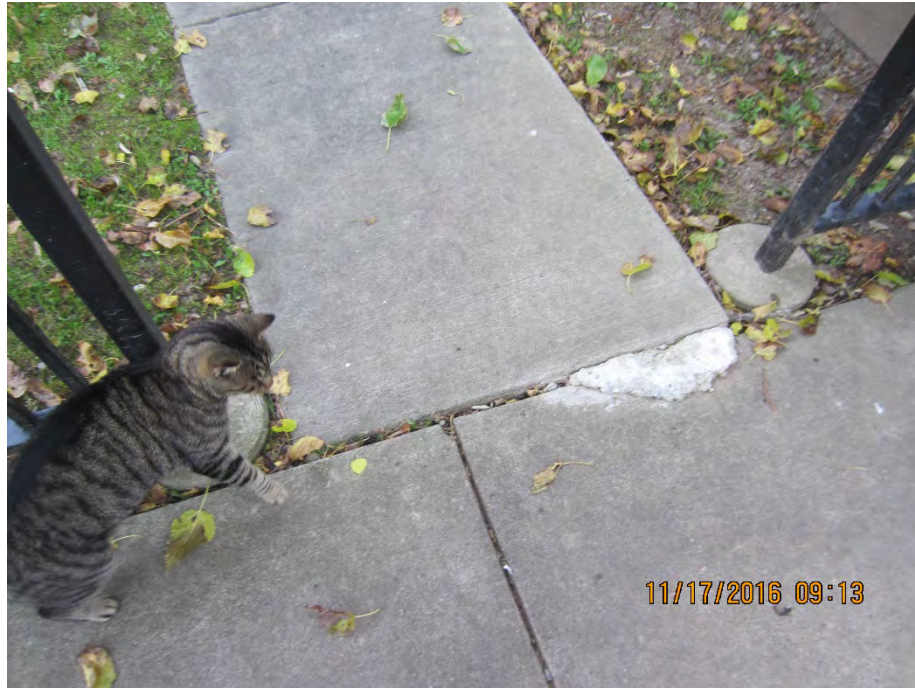
Photo 36 – Replace completely heaved sidewalk [Plan Sheet SP-3]
