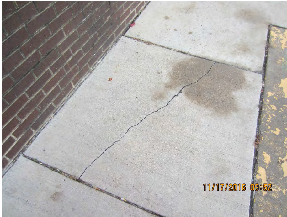
Photo 68a –Clean and seal crack [Plan Sheet SP-5]
