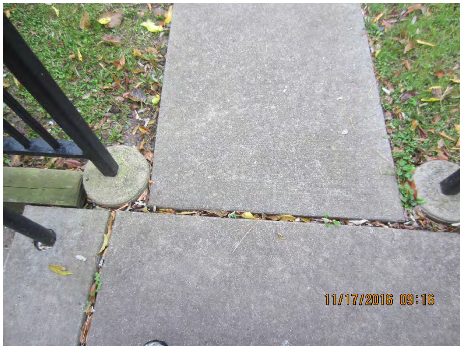
Photo 39 – Foam lift slab & neoprene joint fill [Plan Sheet SP-3]
