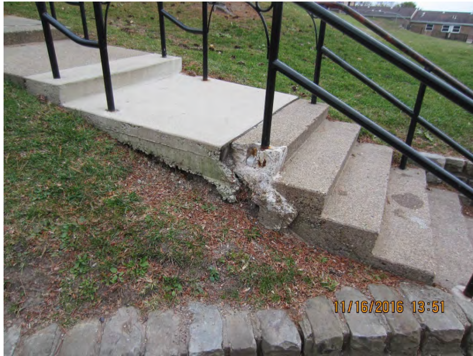
Photo 89 – Repair spalled concrete on steps [Plan Sheet SP-7]
