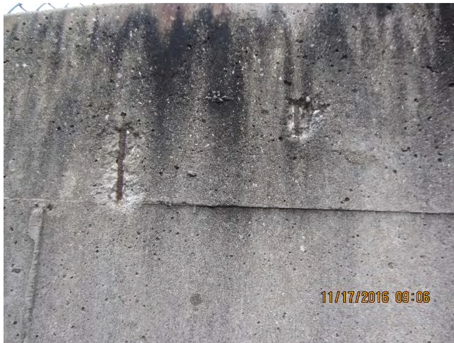
Photo 31 – Repair exposed rebar [Plan Sheet SP-3]
