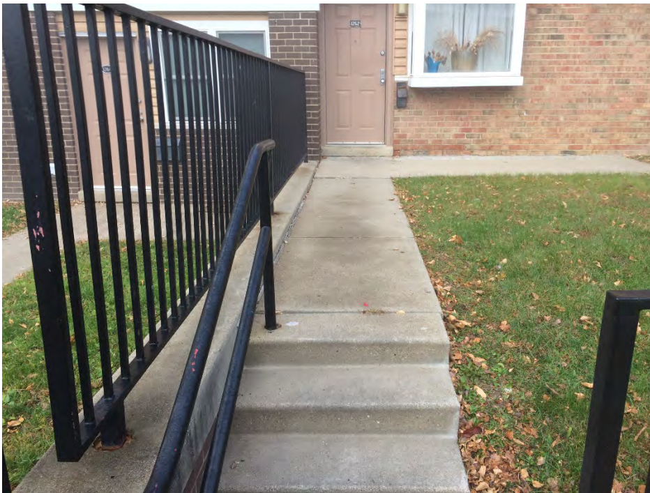
Photo 68 – Neoprene pad crack fill between sidewalk and brick wall [Plan Sheet SP-5]
