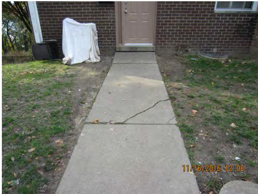
Photo 10d – Replace section of sidewalk [Plan Sheet SP-2]
