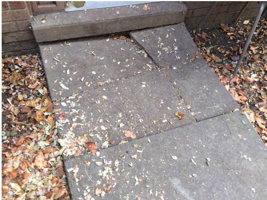
Photo 62 – Remove and replace slab [Plan Sheet SP-4]
