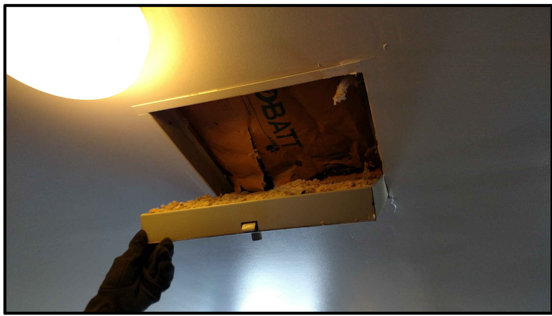
1310 FERRIS LOCATION SMALL ACCESS PANEL INACCESSIBLE 12
