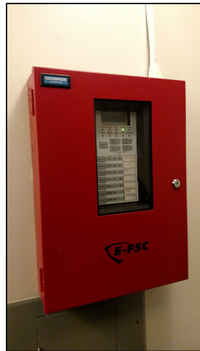
TYPICAL FA MONITORING PANEL 7
