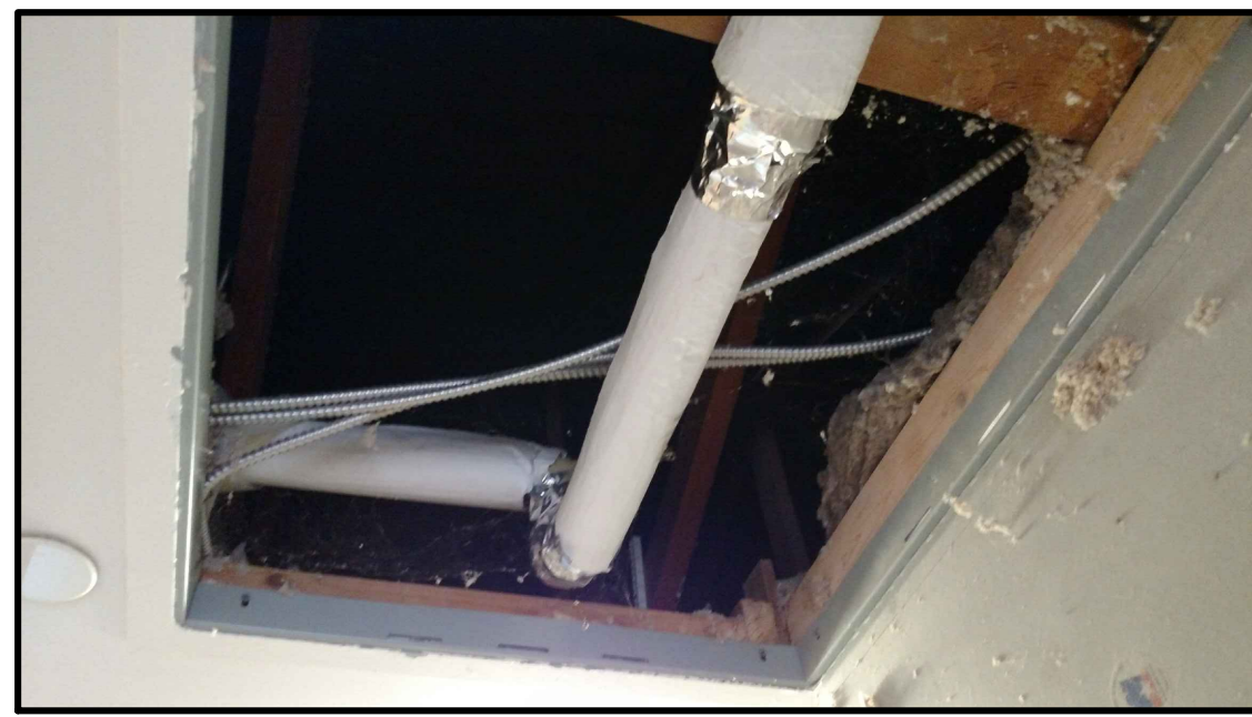
1310 FERRIS LOCATION ACCESS HATCH AND SPRINKLER PIPING 11
