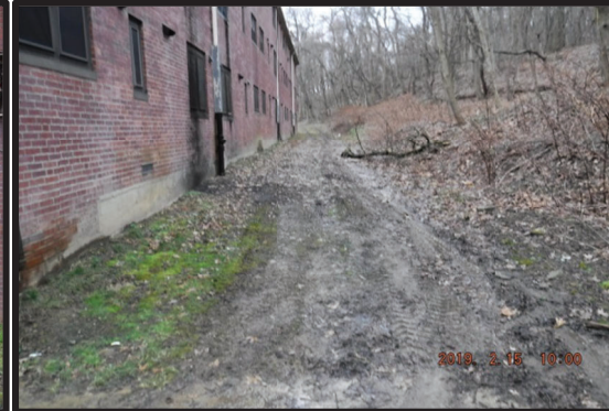
Rear of Bldg. 26
