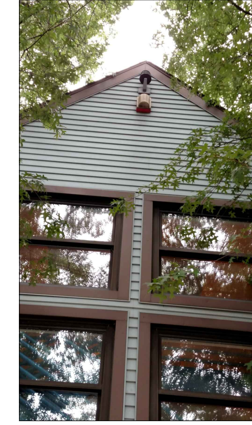
EXISTING BLUE BEACON PICTURE 2 TYPICAL INSTALLATION
