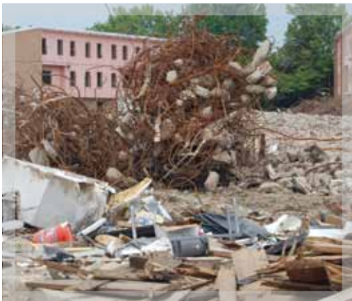
Demolition activity began on site in Addison Terrace in Spring 2013.
