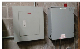
AUXILIARY EM PANEL and SUMP PUMP PANEL
