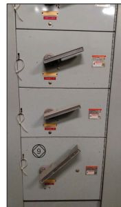
SWITCHBOARD SECTION WITH GENERATOR FEED
