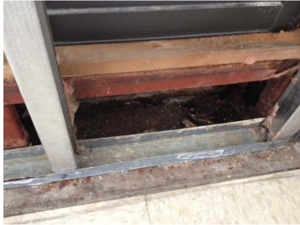
EX. DETERIORATED COLD METAL FRAMING @ WINDOW
