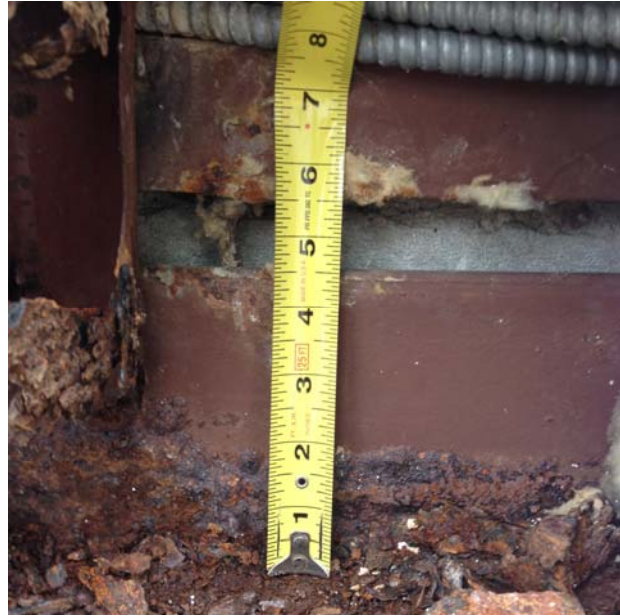
EX. DETERIORATED PLASTER AT CONCRETE PLANKS
