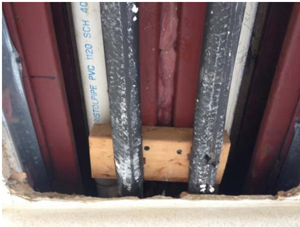
EX. INSULATED PIPING WITHIN FRAMING
