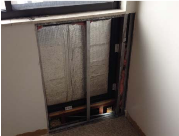
EX. WINDOW SYSTEM FRAMING
