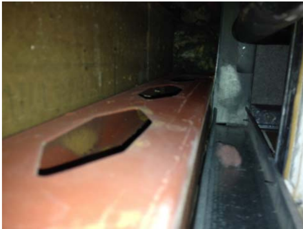
EX. FRAMING EXTENDING PAST CONCRETE PLANK FLOOR
