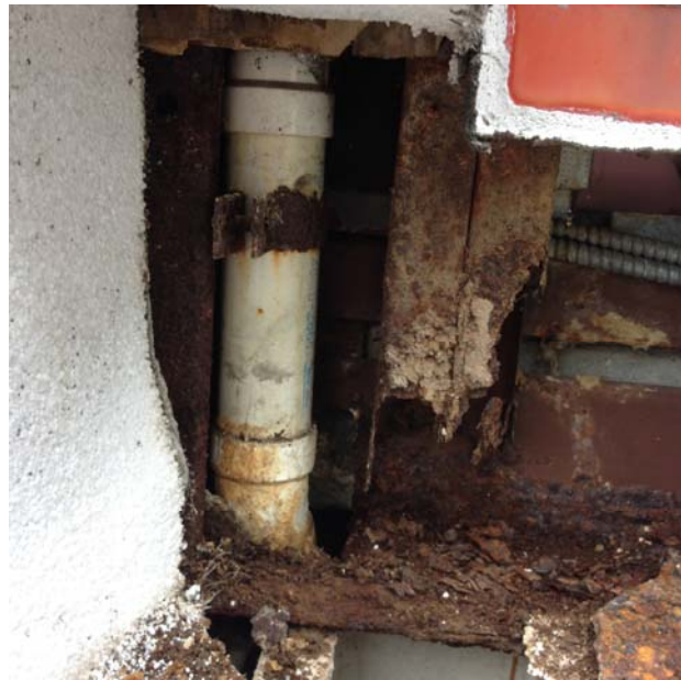
EX. DRAIN PIPE THROUGH PLATES
