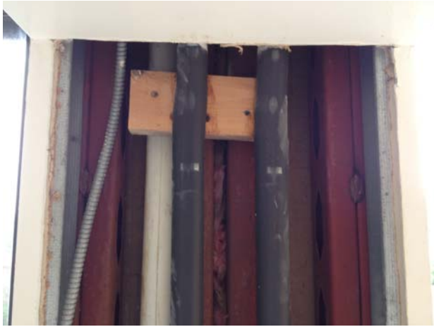
EX. INSULATED PIPING @ KITCHEN SINK
