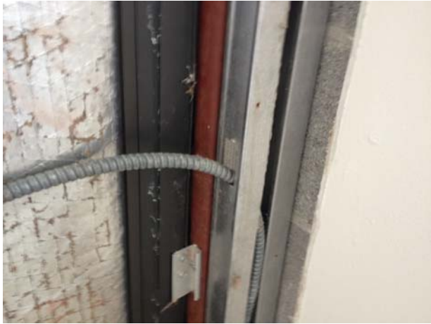
EX. CONDUIT @ METAL FRAMING BELOW WINDOW
