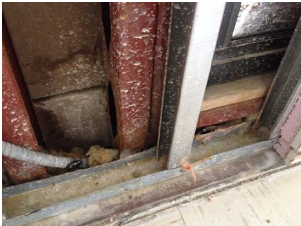
EX. FRAMING/INSULATION AND COLD METAL BEYOND
