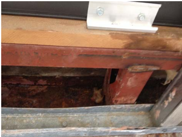
EX. DETERIORATED COLD METAL FRAMING @ WINDOW
