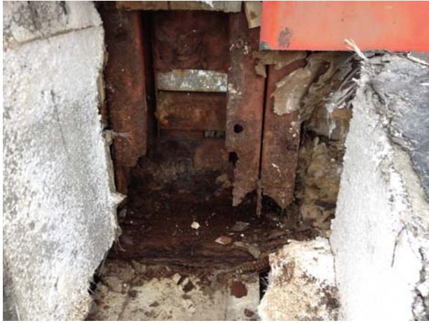
EX. DETERIORATED STEEL PLATES @ MASONRY BASE
