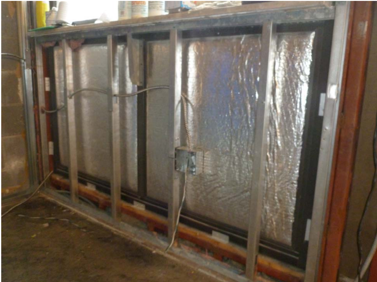
TYPICAL INTERIOR METAL FRAMING AND COLD FORMED METAL FRAMING BELOW WINDOW
