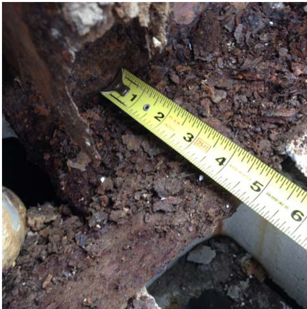
EX. DETERIORATED COLD FORMED METAL FRAMING
