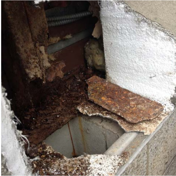
EX. DETERIORATED STEEL PLATES @ MASONRY BASE
