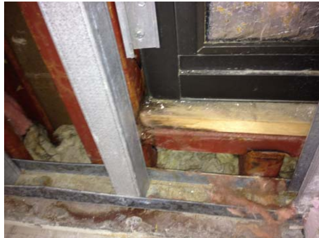
EX. INTERIOR FRAMING AND COLD METAL BEYOND
