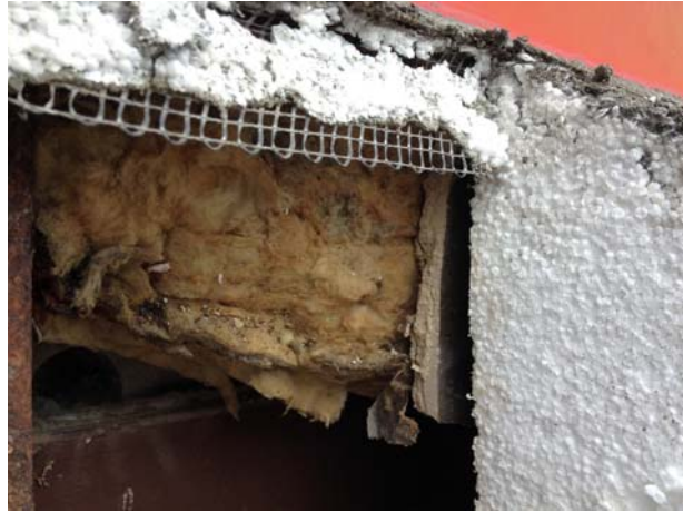
EX. WATER DAMAGED BATT INSULATION
