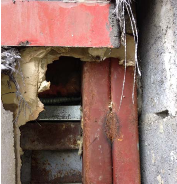
EX. STEEL ANGLES AT CONCRETE PLANKS
