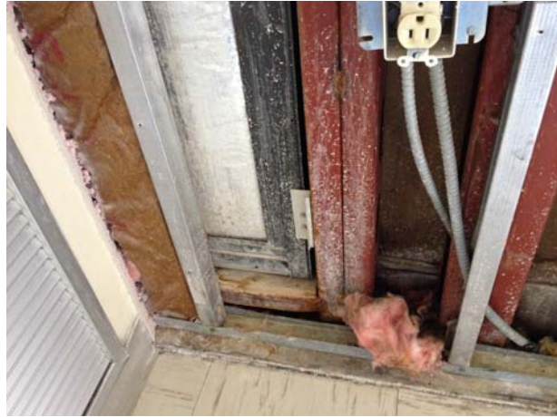
EX. WINDOW SYSTEM SECURED TO METAL FRAMING
