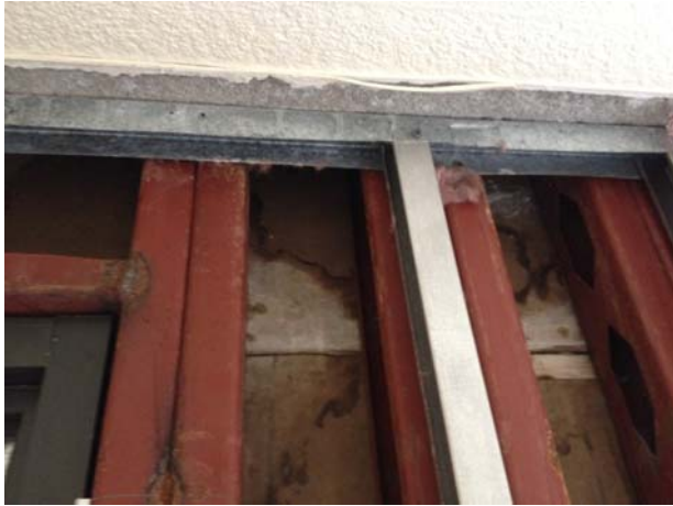
EX. COLD FORMED METAL FRAMING
