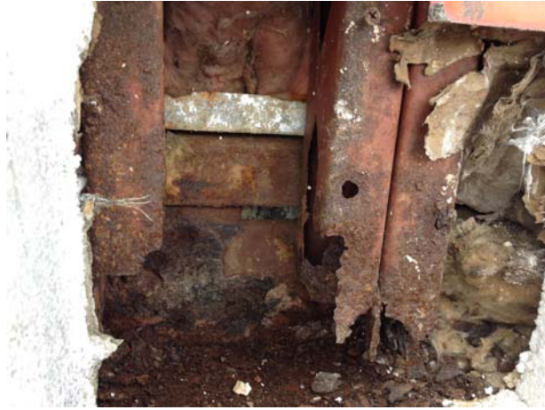
EX. DETERIORATED COLD FORMED METAL FRAMING
