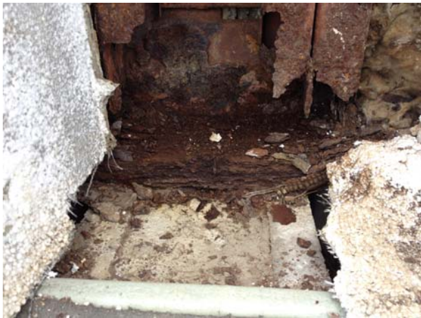
EX. MASONRY CELLS - PARTIALLY GROUTED
