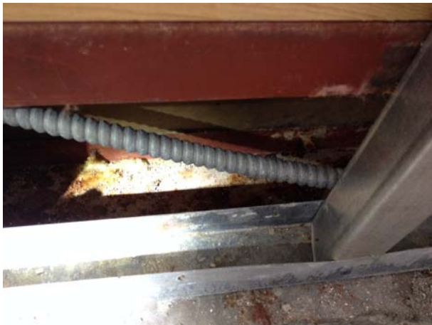
EX. DETERIORATED COLD METAL FRAMING @ WINDOW
