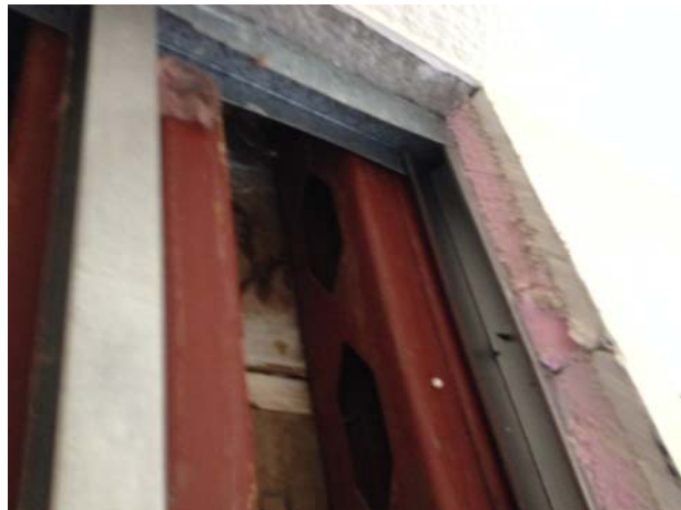
EX. FRAMING/INSULATION AND COLD METAL BEYOND
