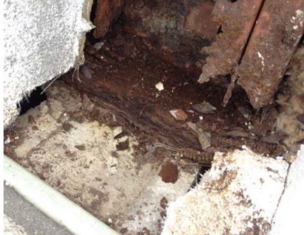
EX. MASONRY CELLS – PARTIALLY GROUTED
