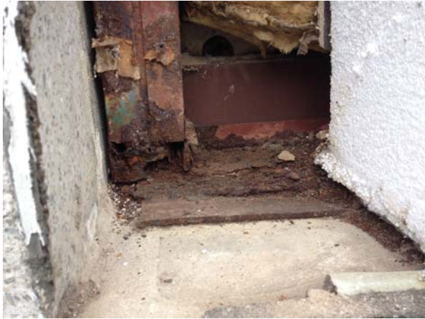
EX. DETERIORATED COLD FORMED METAL FRAMING
