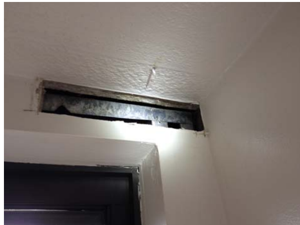
EX. VIEW OF FRAMING ABOVE WINDOW
