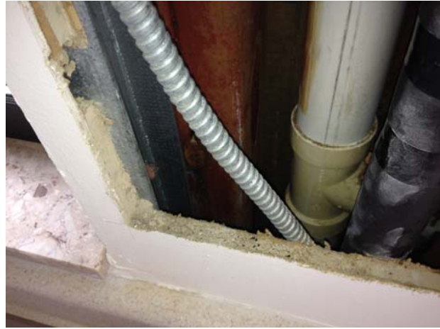
EX. CONDUIT WITHIN METAL FRAMING
