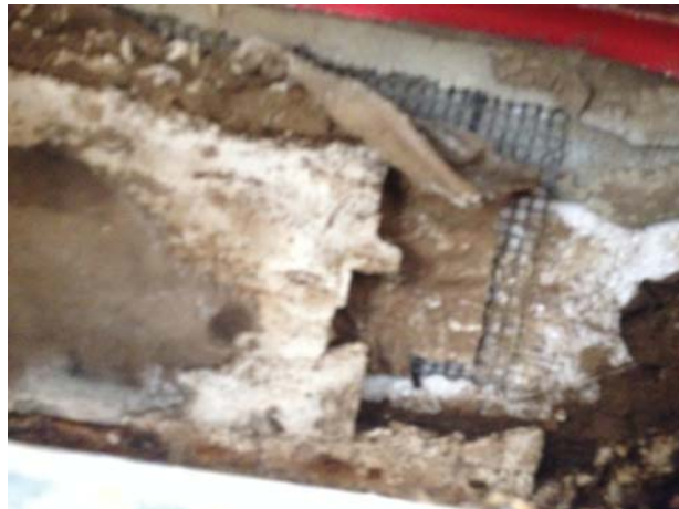
EX. DETERIORATED EIFS BELOW WINDOW
