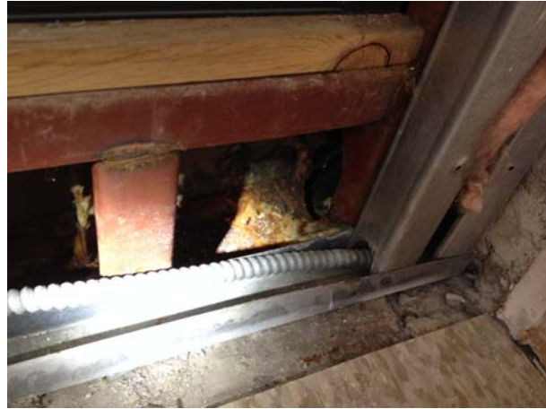
EX. DETERIORATED COLD METAL FRAMING @ WINDOW
