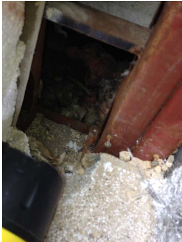
EX. BETWEEN CONCRETE PLANK AND MASONRY BASE
