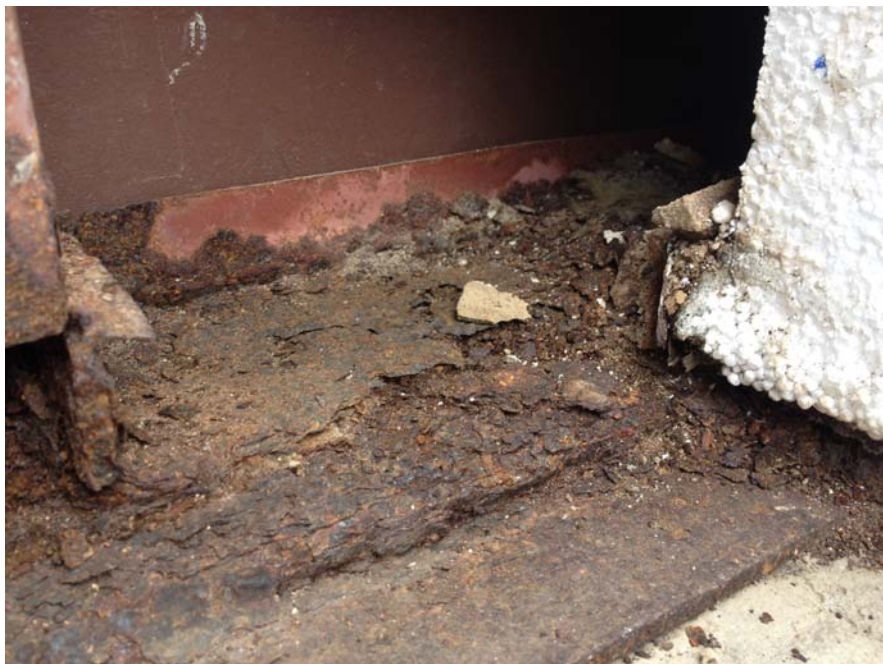
EX. DETERIORATED STEEL PLATES @ MASONRY BASE
